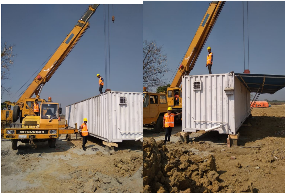
10 Mar 2020 : Container Office Installation
