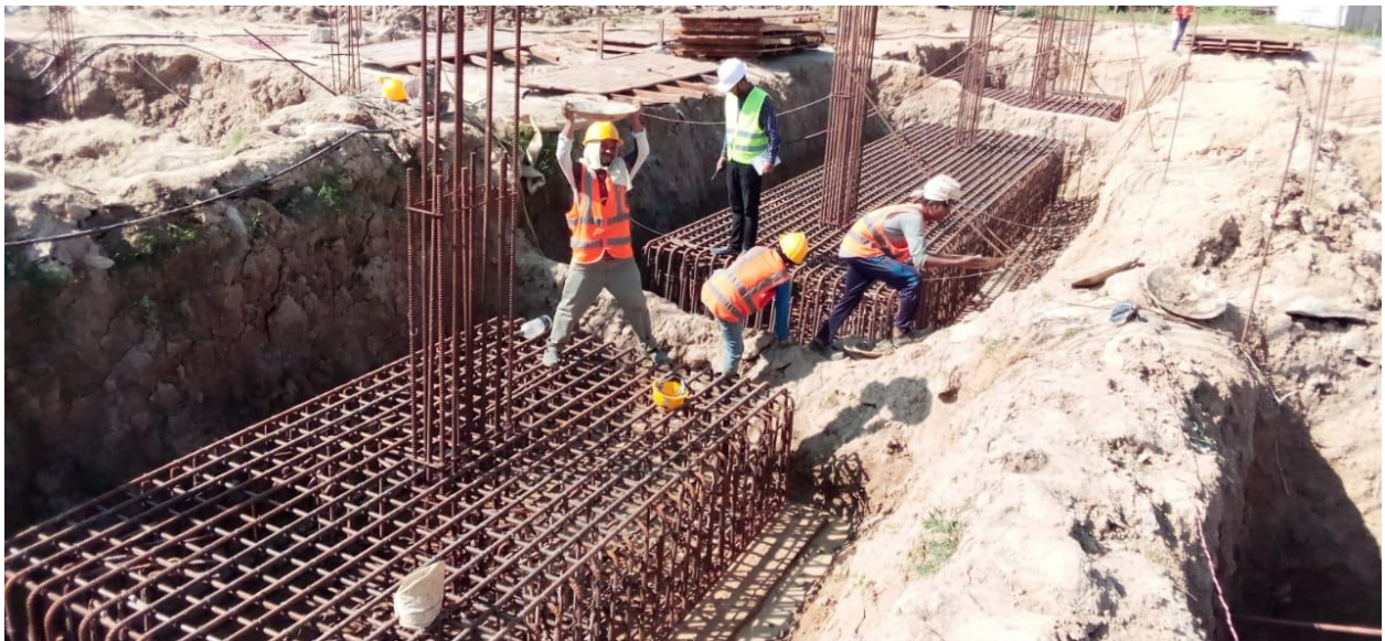
11-14 Nov 2020 : Pile cap Re-bar work
