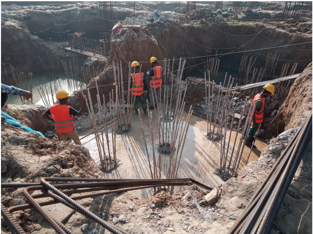
07 Nov 2020: Pile Cap preparation
