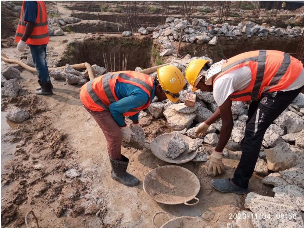
04 Nov 2020: Pile head breaking
