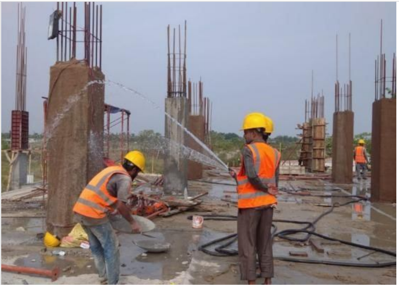
Column Curing on 09-05-21
