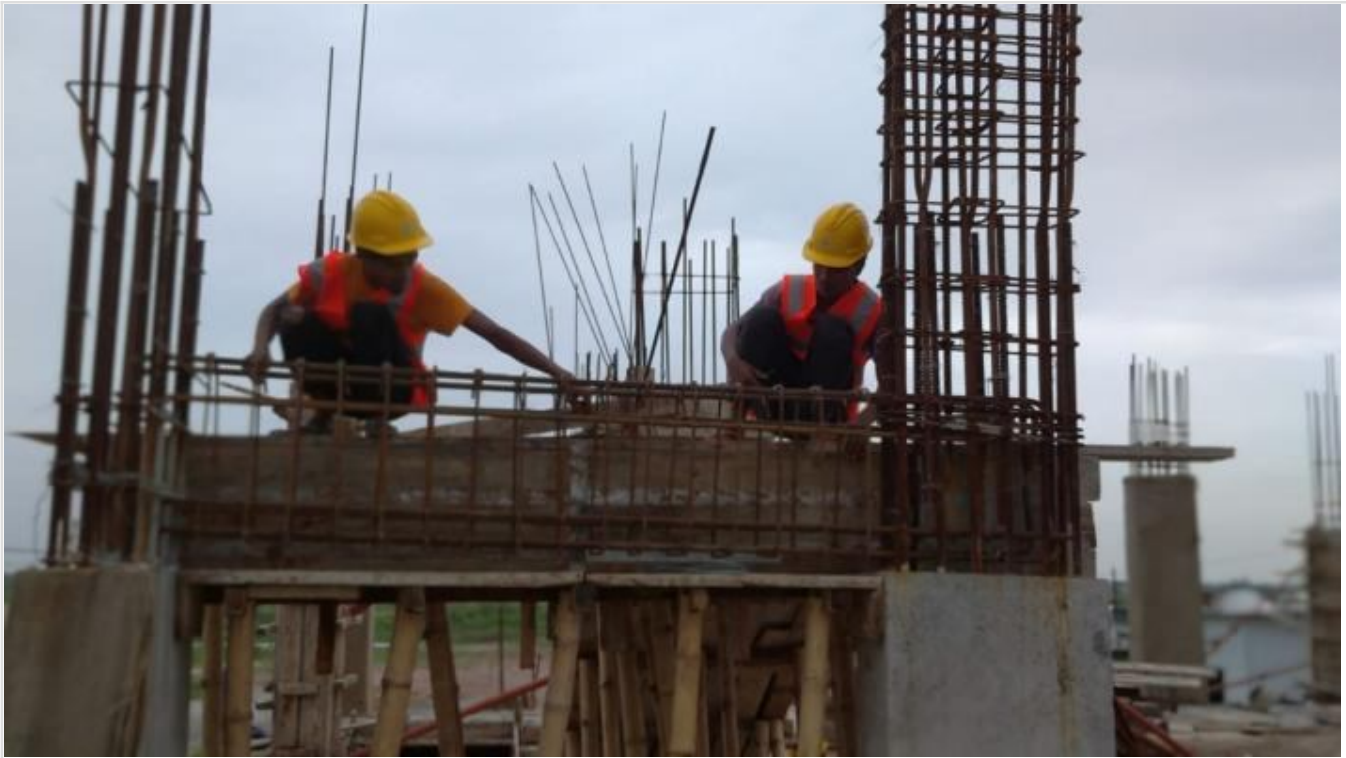
Ground Floor-Roof Beam Shuttering on 26-05-21
