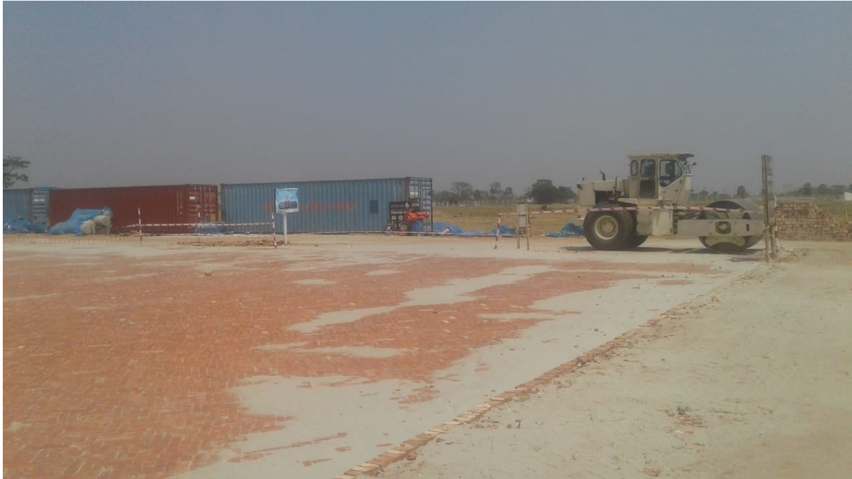
28 Mar 2020: Lay-down Area
