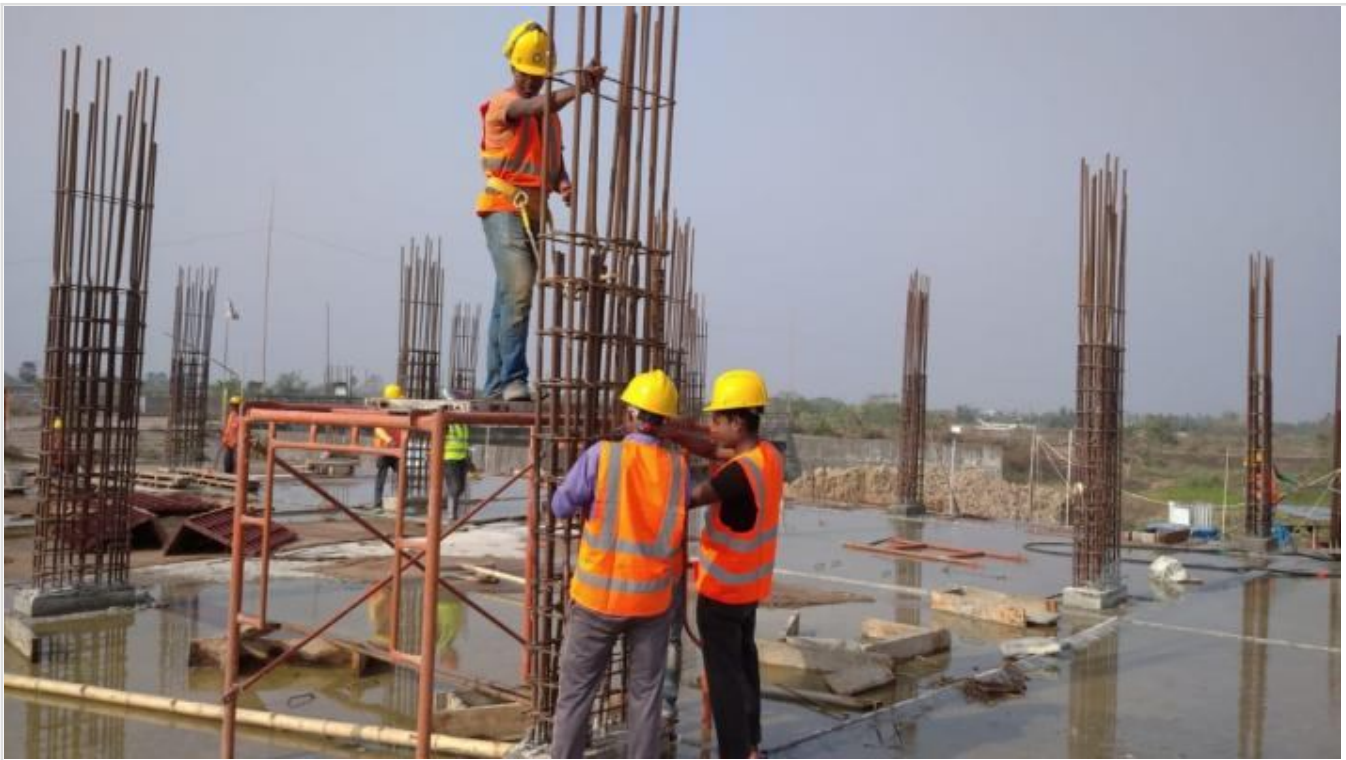
Ground Floor Column Re-bar Work on 01-04-21
