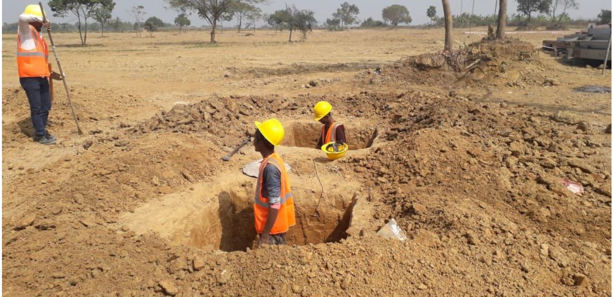
10 Feb 2020: Excavation for Boundary Wall Footing
