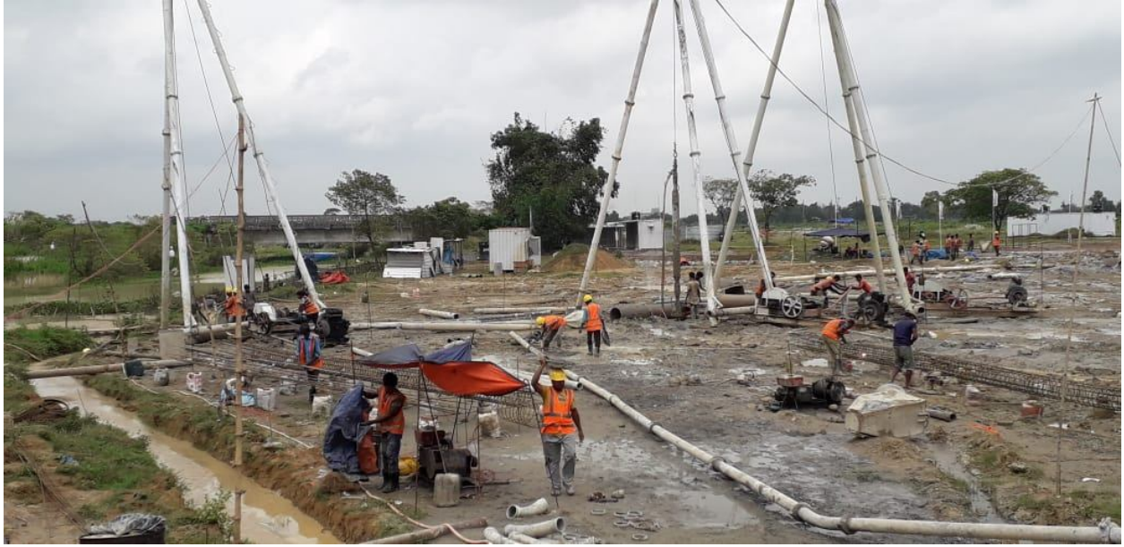
23 Sep 2020: Sales Office Piling Work
