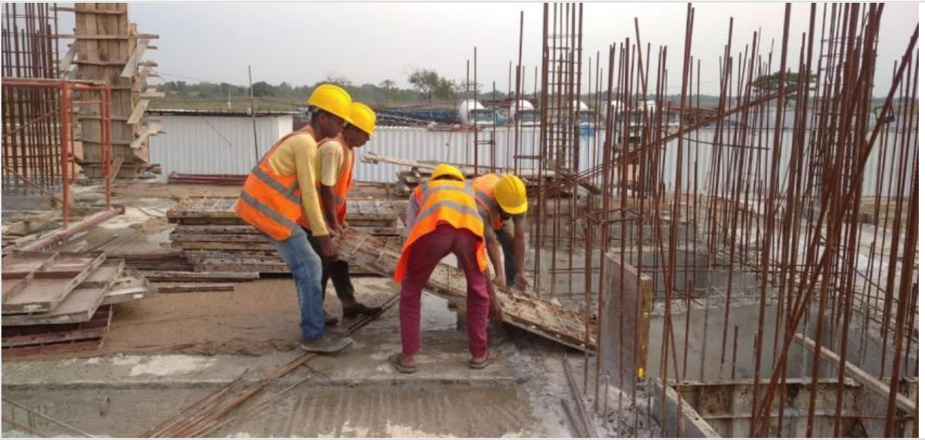
Column Shuttering Work on 08-05-21
