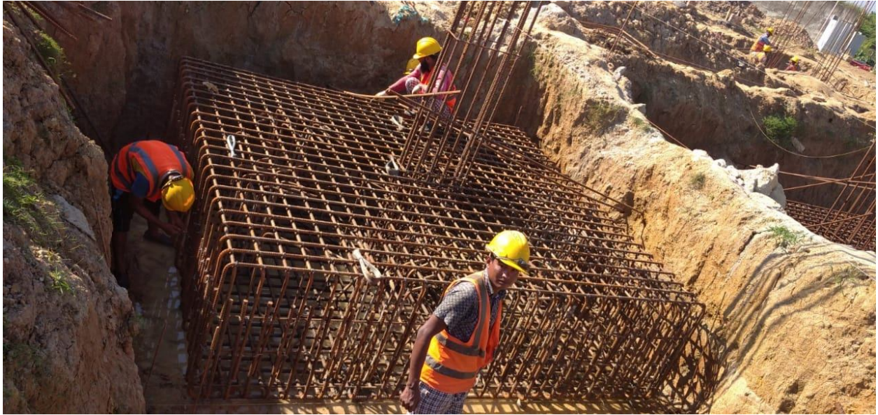
11-14 Nov 2020 : Pile cap Re-bar work
