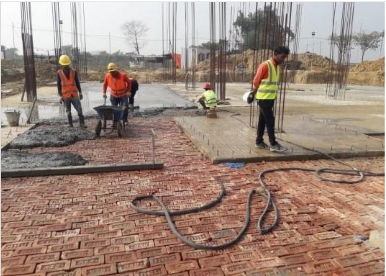
Mat CC Concreting on 15-12-20
