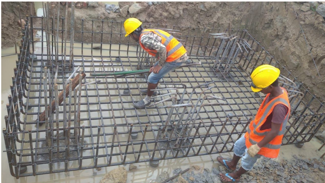
31 Oct 2020 : Pile Cap Re-bar work
