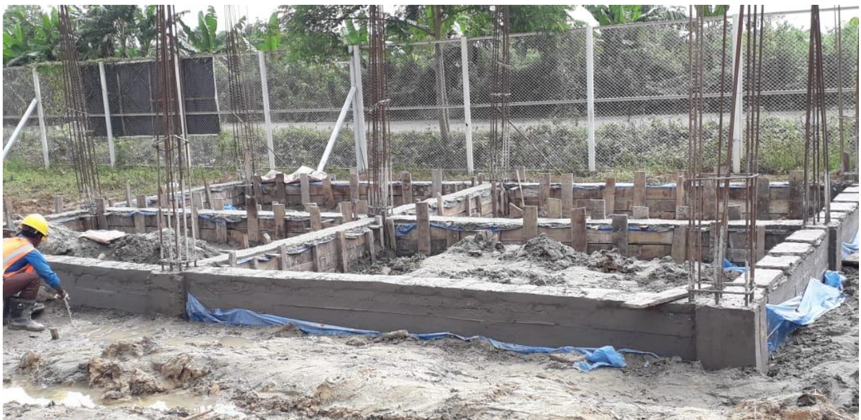
23 Sep 2020: Substation Grade beam
