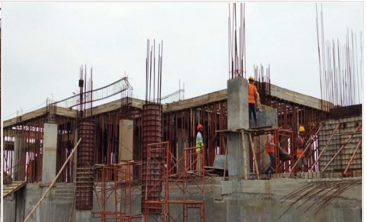
Ground Floor Construction on 07-06-21
