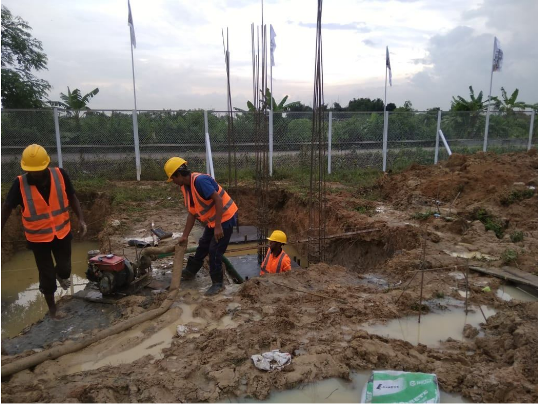
13 Sep 2020 : Sub-station Footing CC
