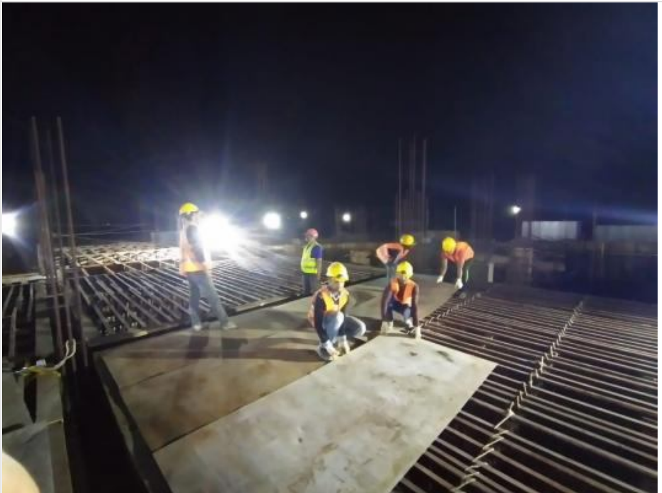
Night Shift Working on 04-03-21
