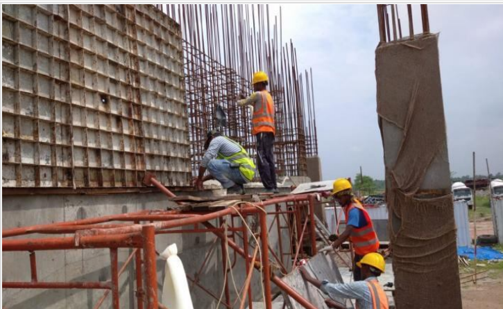
Ground Floor Lift Core Shuttering on 15-06-21
