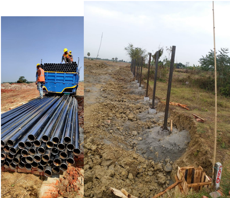
03 Mar 2020: Boundary Fencing Column
