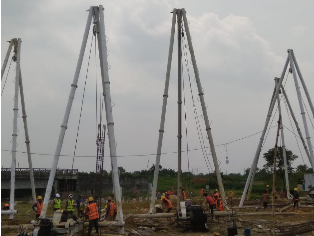
30 Aug 2020: Piling Work
