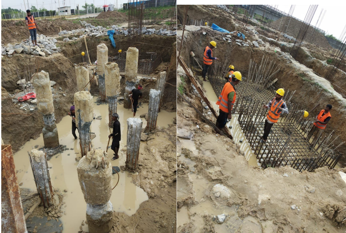
03-04 Nov 2020 : Pile Head Breaking, Pile cap re-bar
