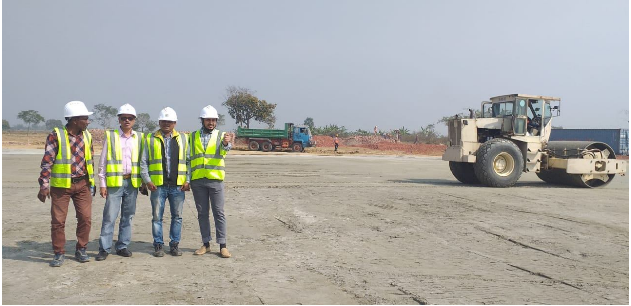
28 Feb 2020: Compaction in Laydown Area
