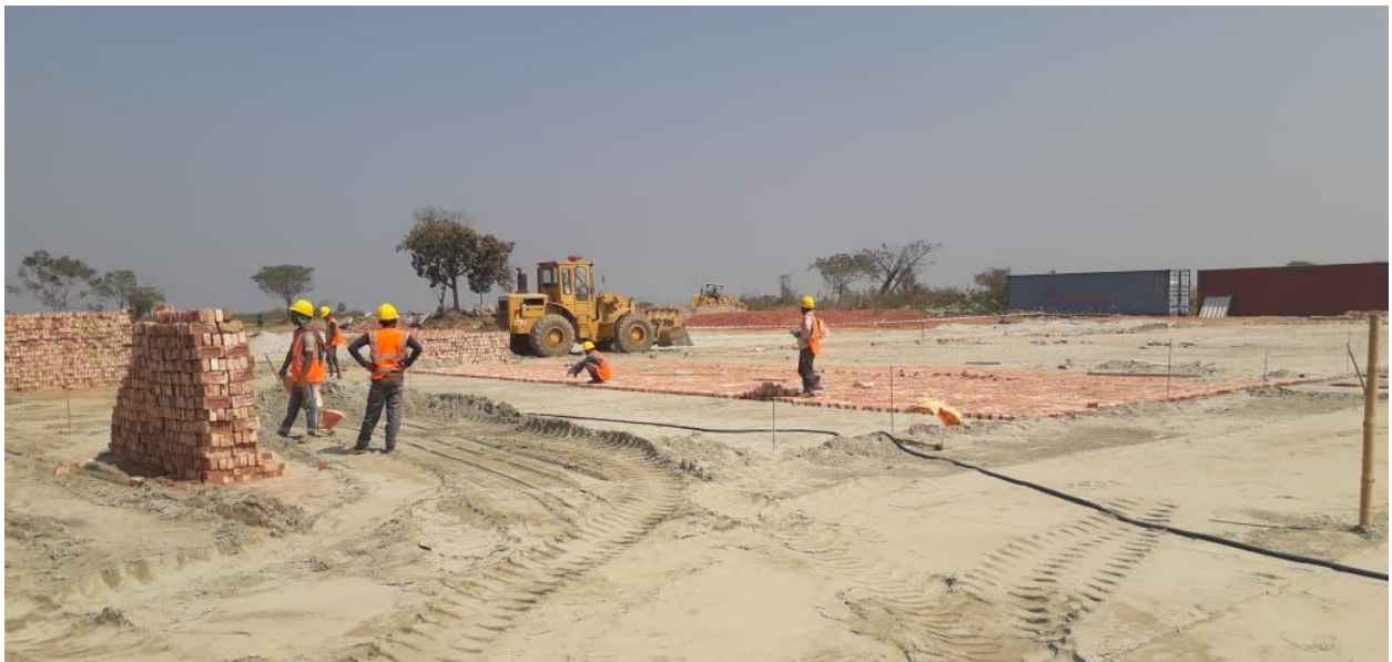
28 Feb 2020: Brick Soling in Laydown Area
