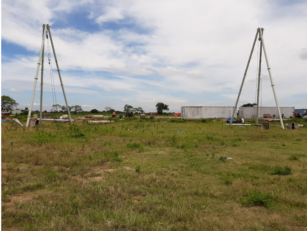
25 Aug 2020: Piling Rig Installed
