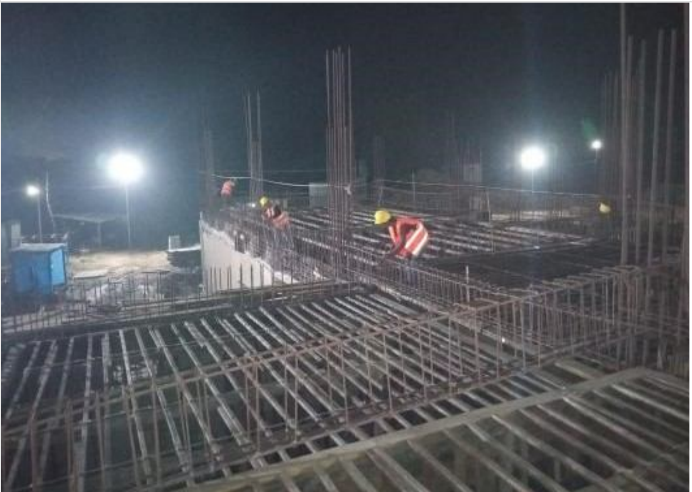
GF Slab Re-bar Work at Night Shift on 08-03-21
