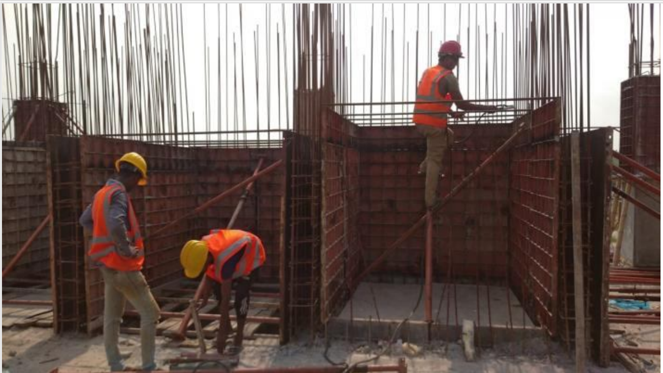
Ground Floor-Lift Wall Shuttering on 30-05-21
