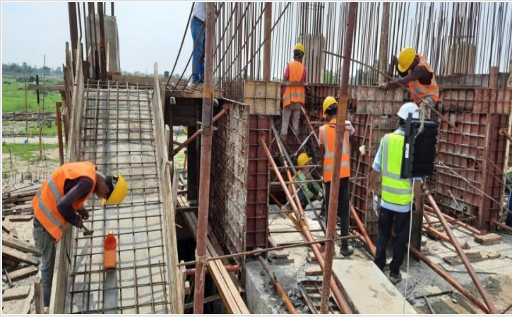
Ground Floor Stair Re-bar work on 09-06-21
