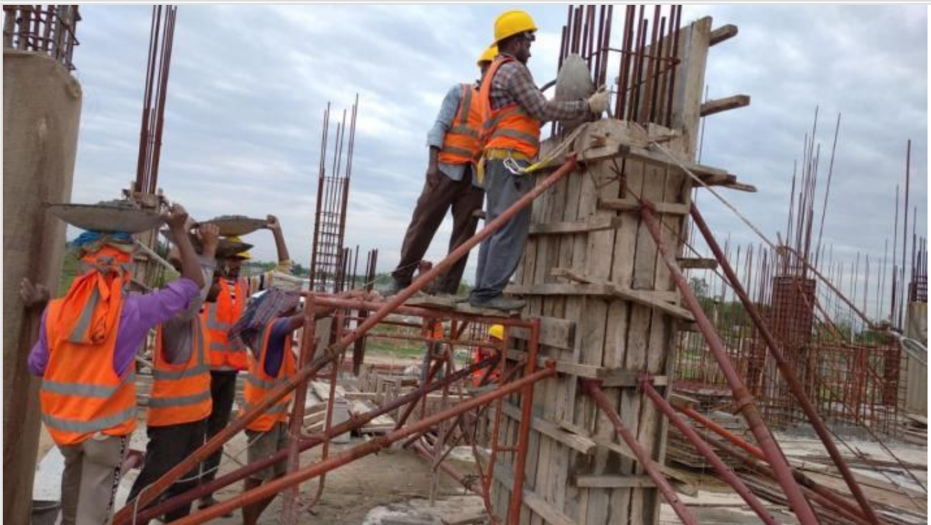
Ground Floor-Column Concreting on 25-05-21
