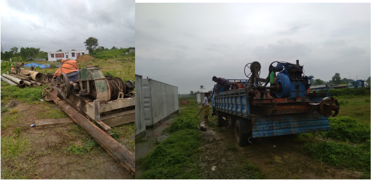
21-22 Aug 2020 : Piling Rig Mobilization for Sales Centre
