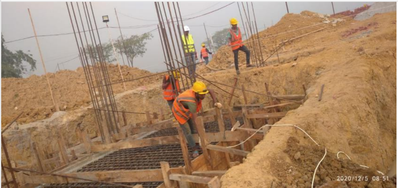
Pile Cap Re-bar Shuttering Work on 05-12-20
