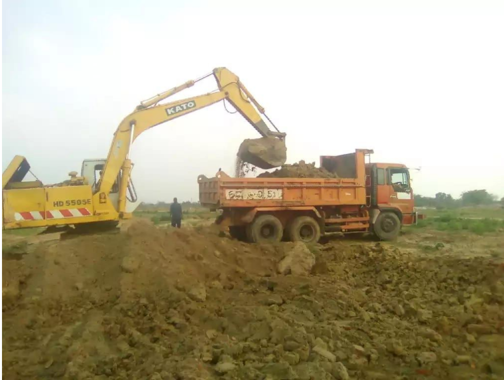
04 May 2020: Earth Loading for Site Development
