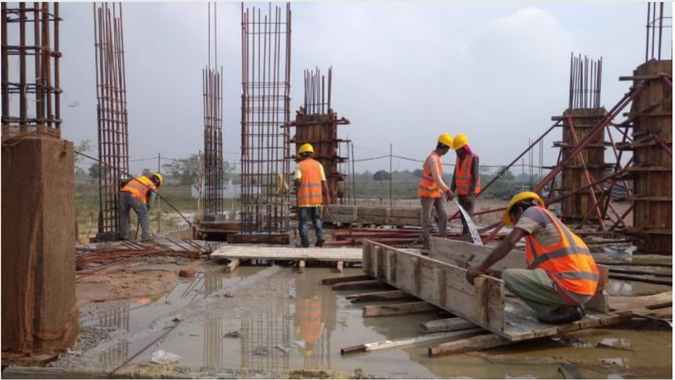
Column Shuttering Work on 04-05-21
