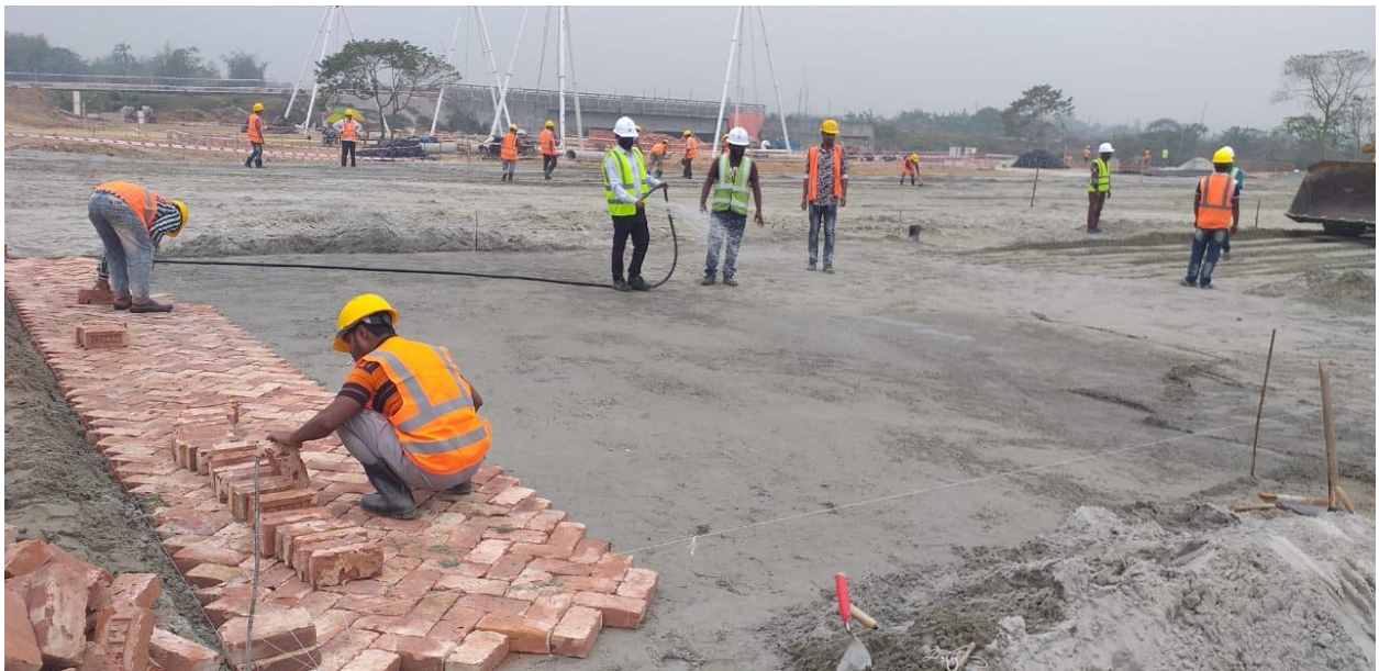
28 Feb 2020: Herring Bone Bond working in Laydown Area
