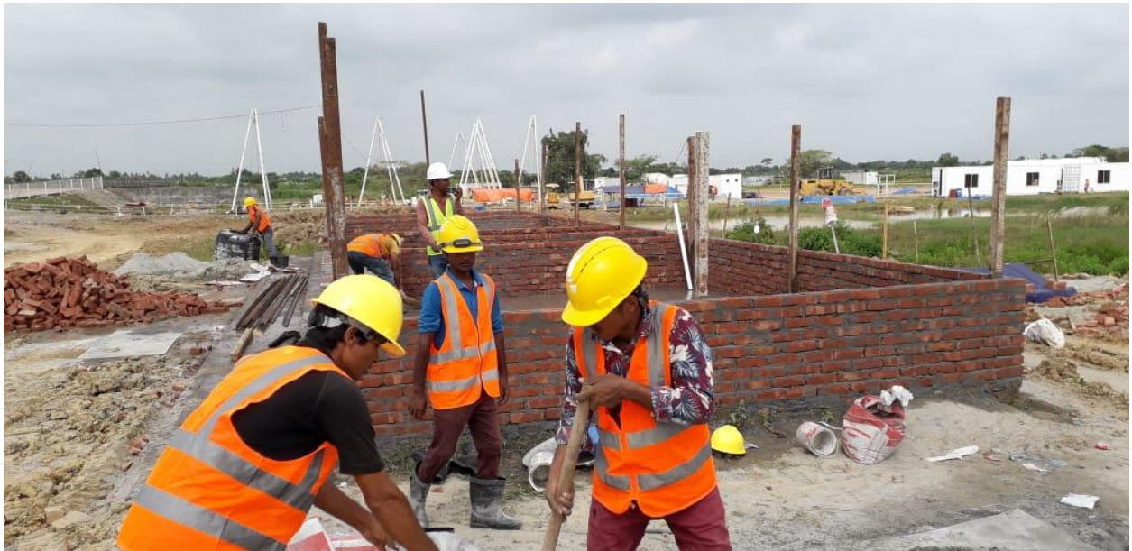
06 Sep 2020: Site Office and Staff Residence
