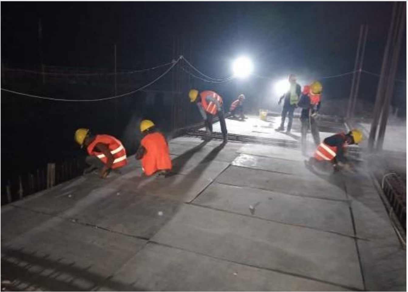
GF Slab Shuttering at Night Shift on 08-03-21
