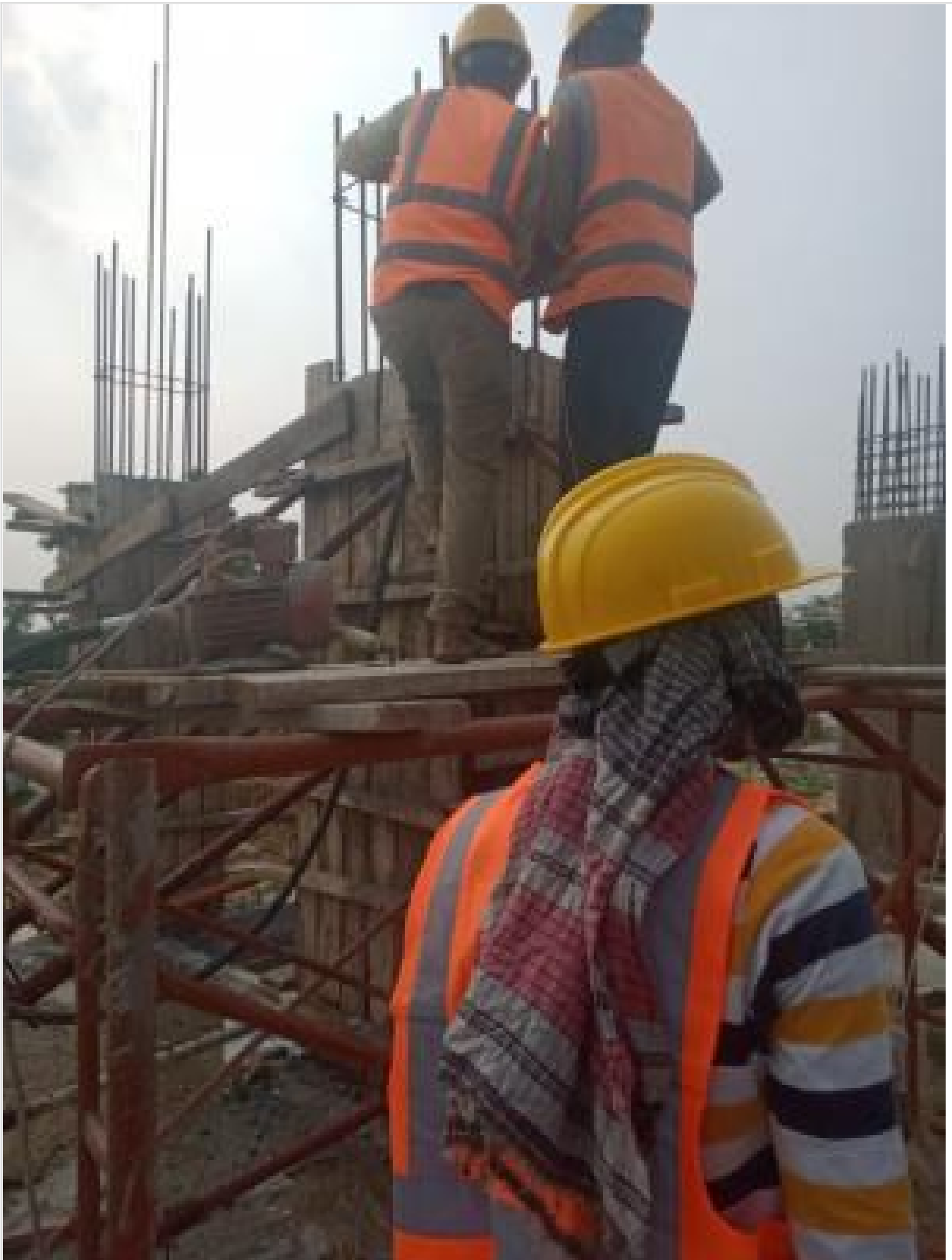
Ground Floor-Column Concreting on 23-05-21
