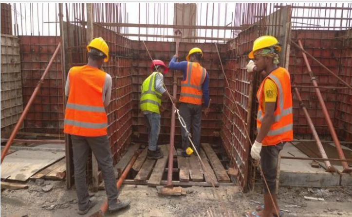
Ground floor Lift Core Shuttering on 07-06-21
