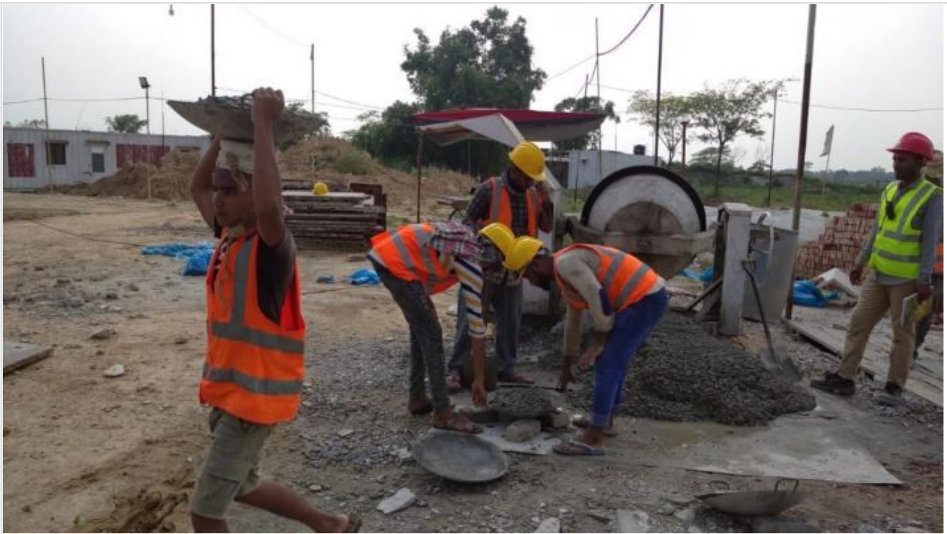
Ground Floor-Column Concreting on 23-05-21
