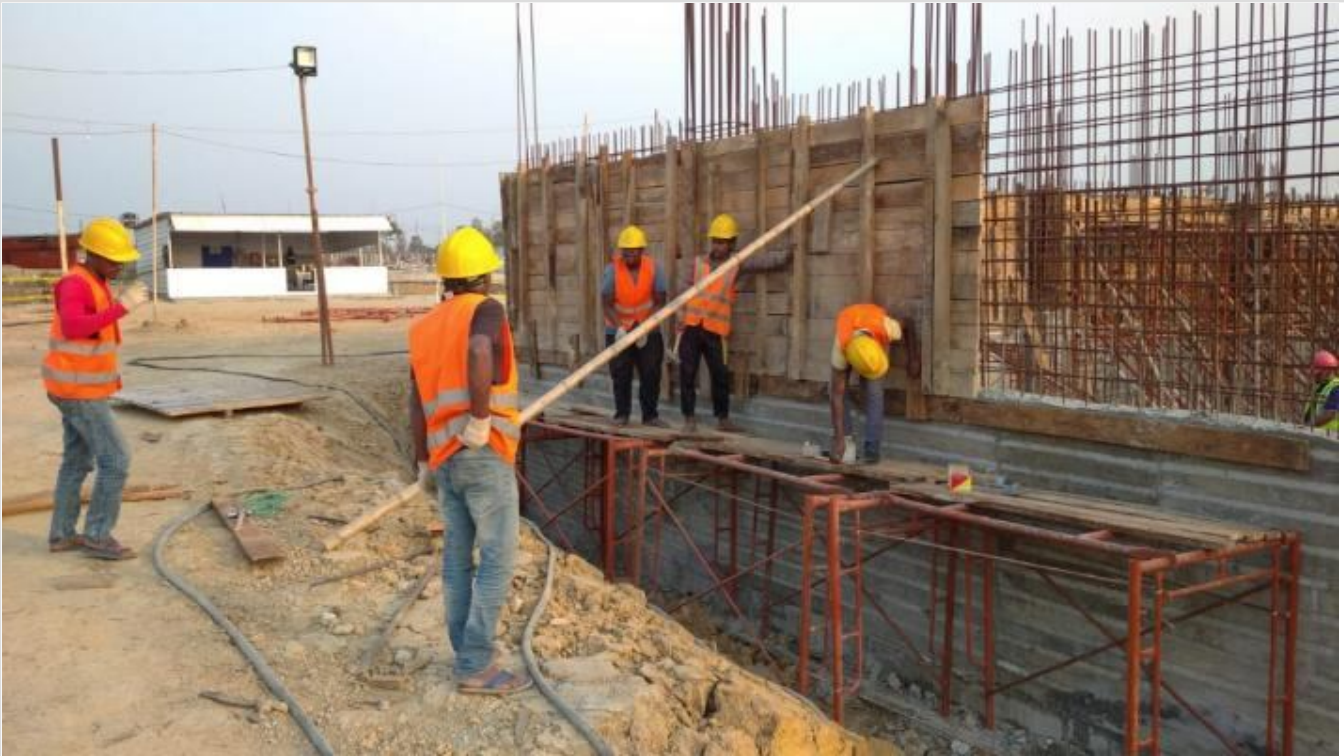
Retaining Wall Shuttering on 18-02-21
