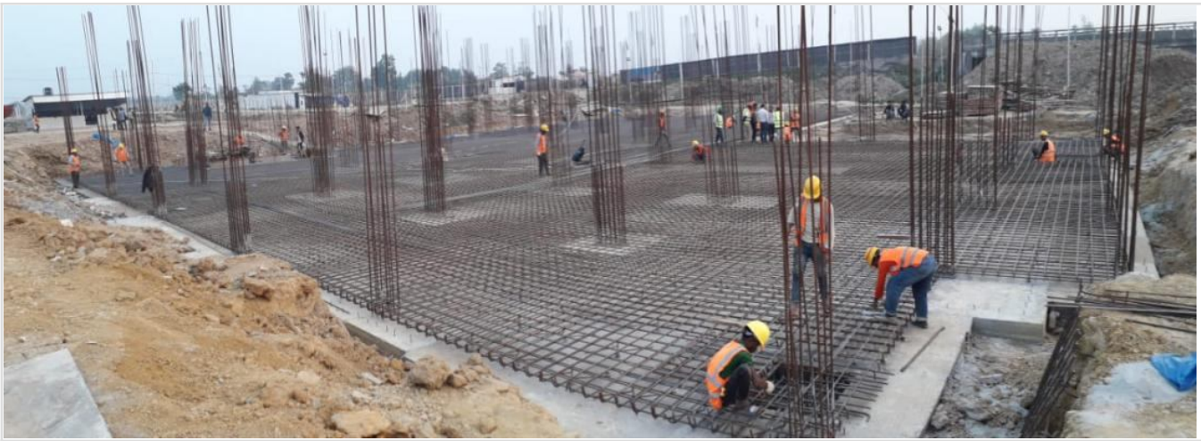
Mat Re-bar Work on 29-12-20
