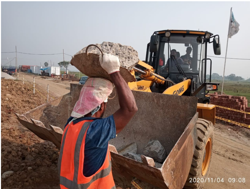
04 Nov 2020: Pile head breaking
