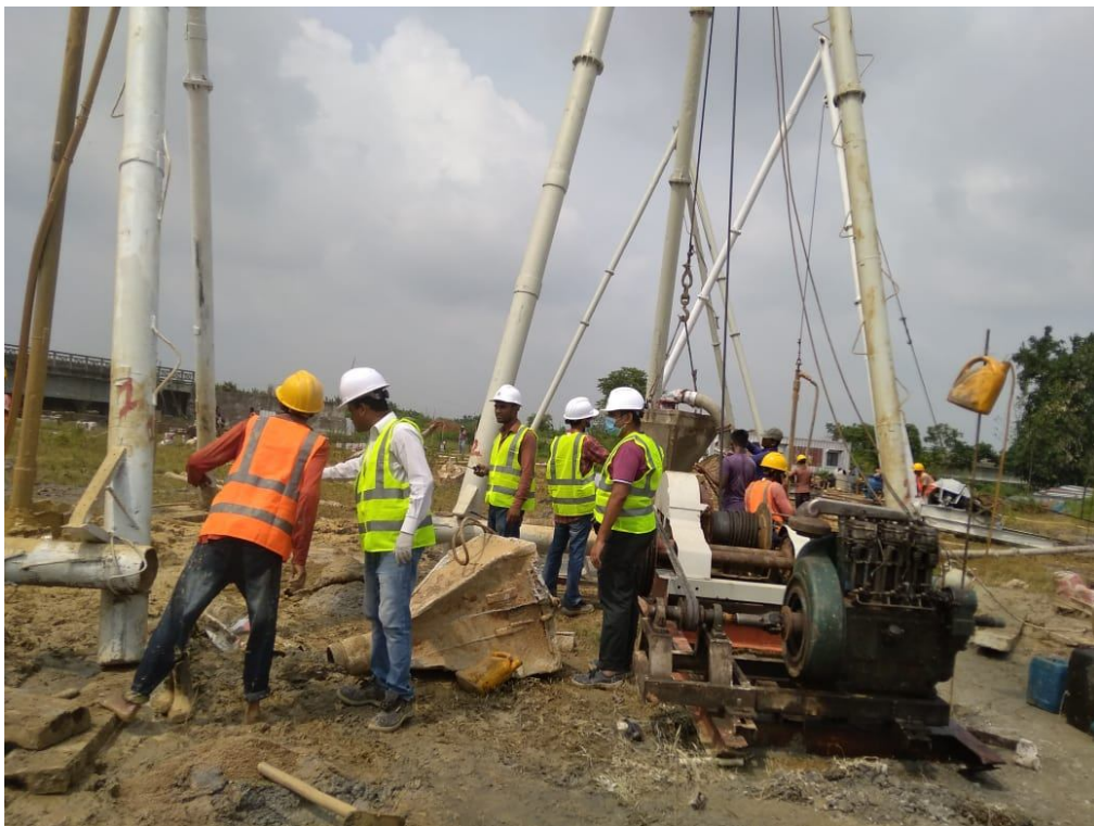
30 Aug 2020: Piling Work
