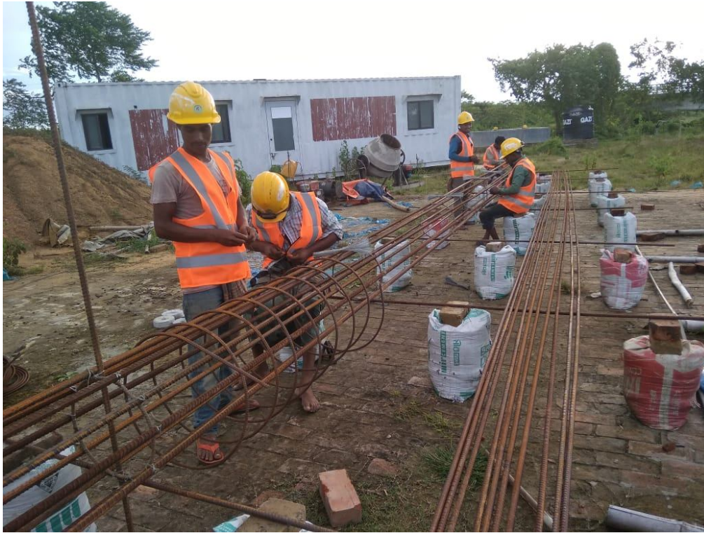
25 Aug 2020: Pile Re-barwork
