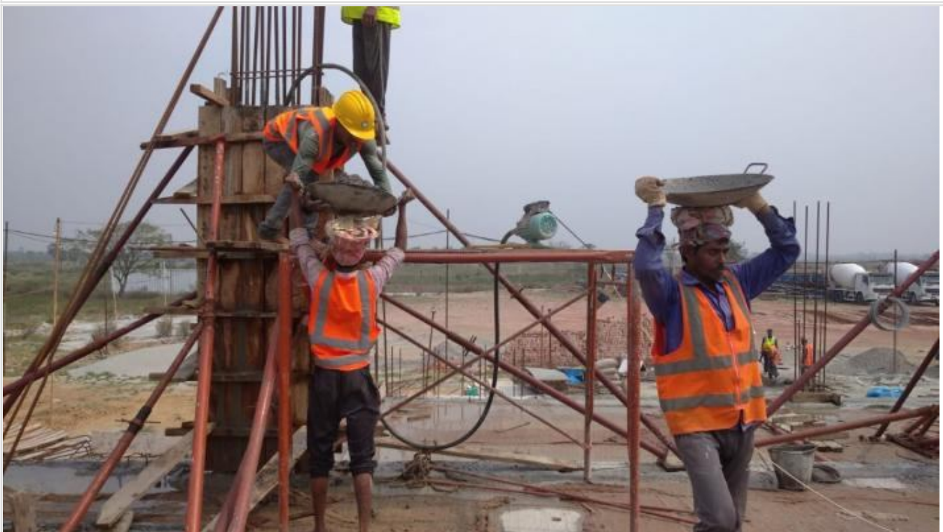
Column Concreting on 03-05-21
