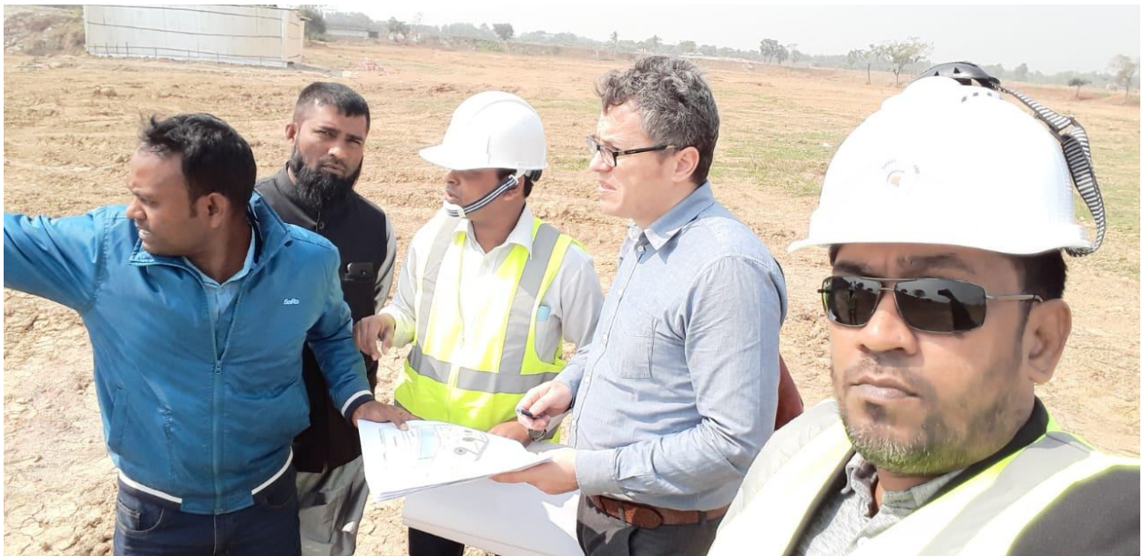
10 Feb 2020 : Layout Inspection
