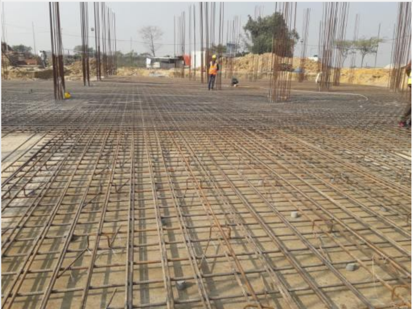
Mat Re-bar Work on 29-12-20
