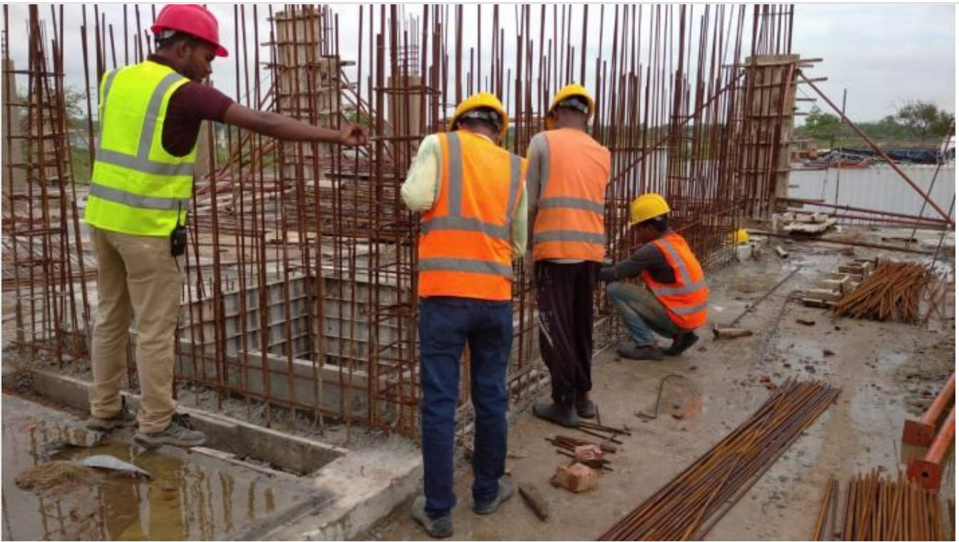
Ground Floor-Lift Core-Re-bar Work on 25-05-21
