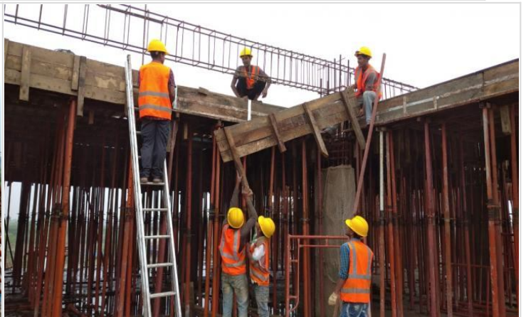
1st Floor Beam Shuttering on 06-06-21
