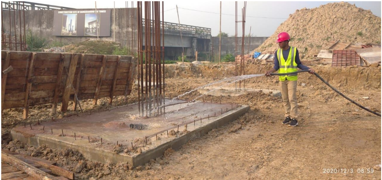
03 Dec 2020 : Concrete curing
