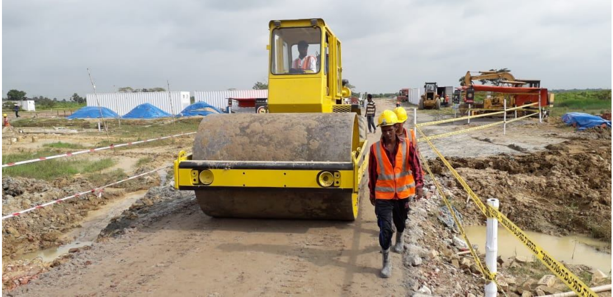
06 Sep 2020: Road Compaction
