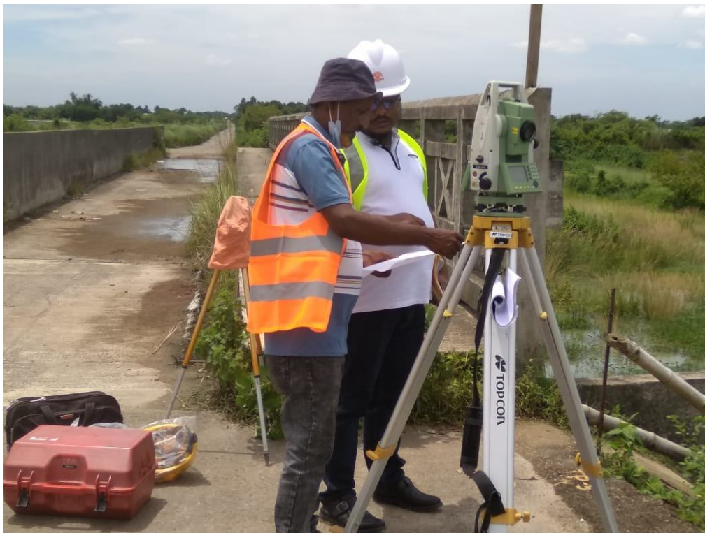
25 Aug 2020: Providing Piling Point
