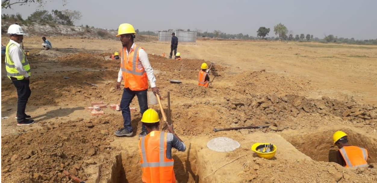
10 Feb 2024 – Excavation for Boundary Fencing Footing
