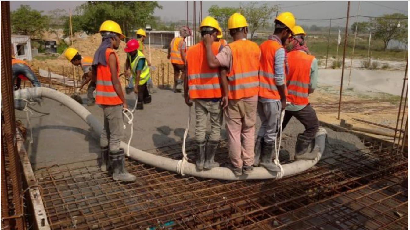
Ground Floor Slab Concreting on 25-04-21
