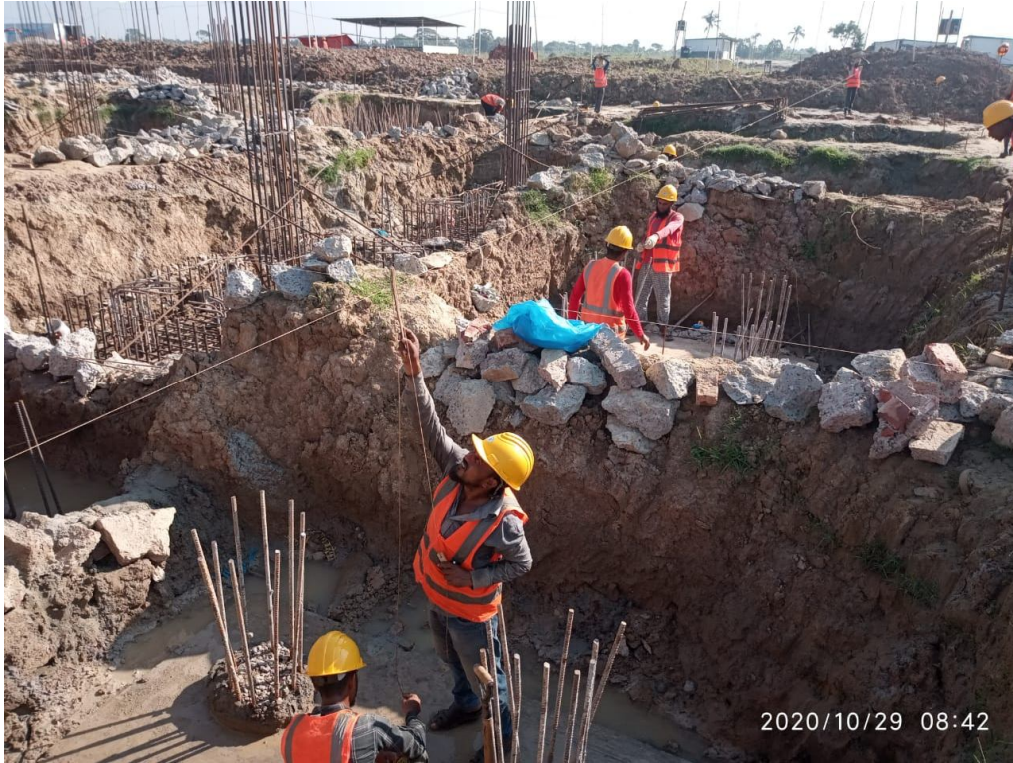
29 Oct 2020: Column Point fixing
