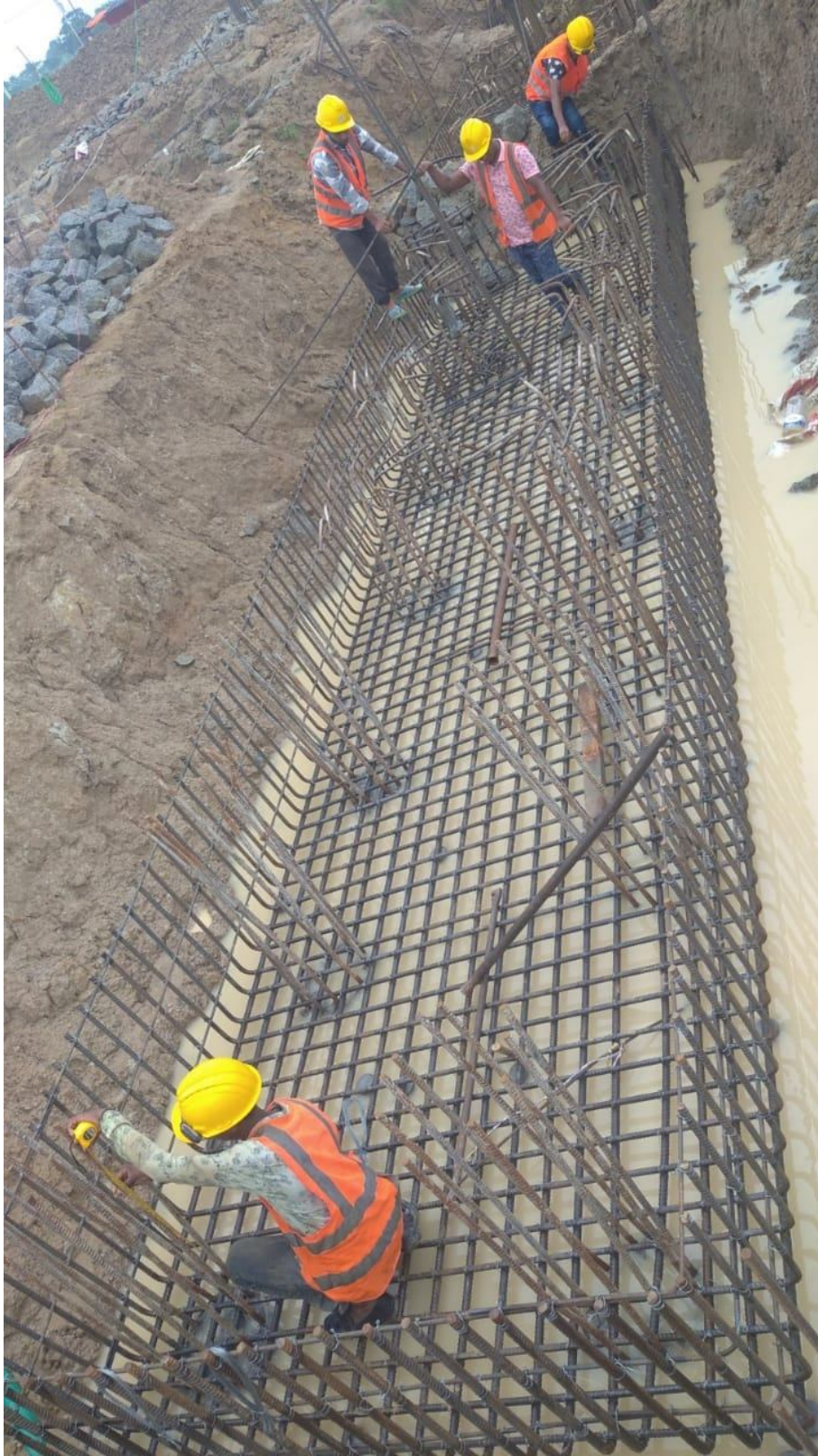
31 Oct 2020 : Pile Cap Re-bar work
