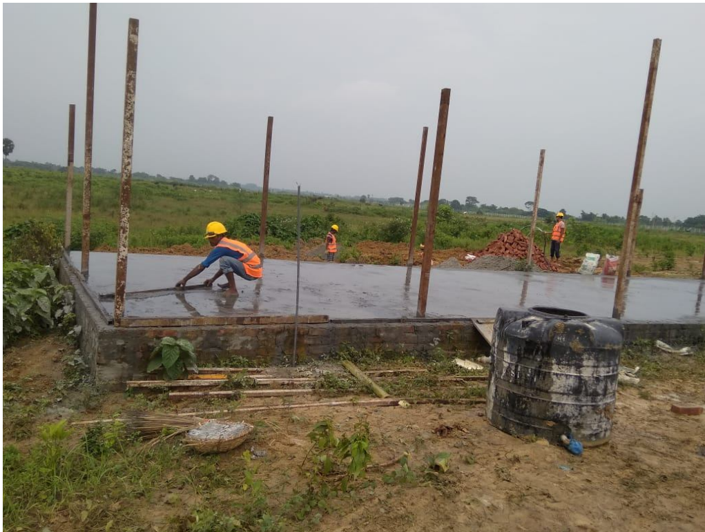
31 Aug 2020: Site Office and Staff Residence
