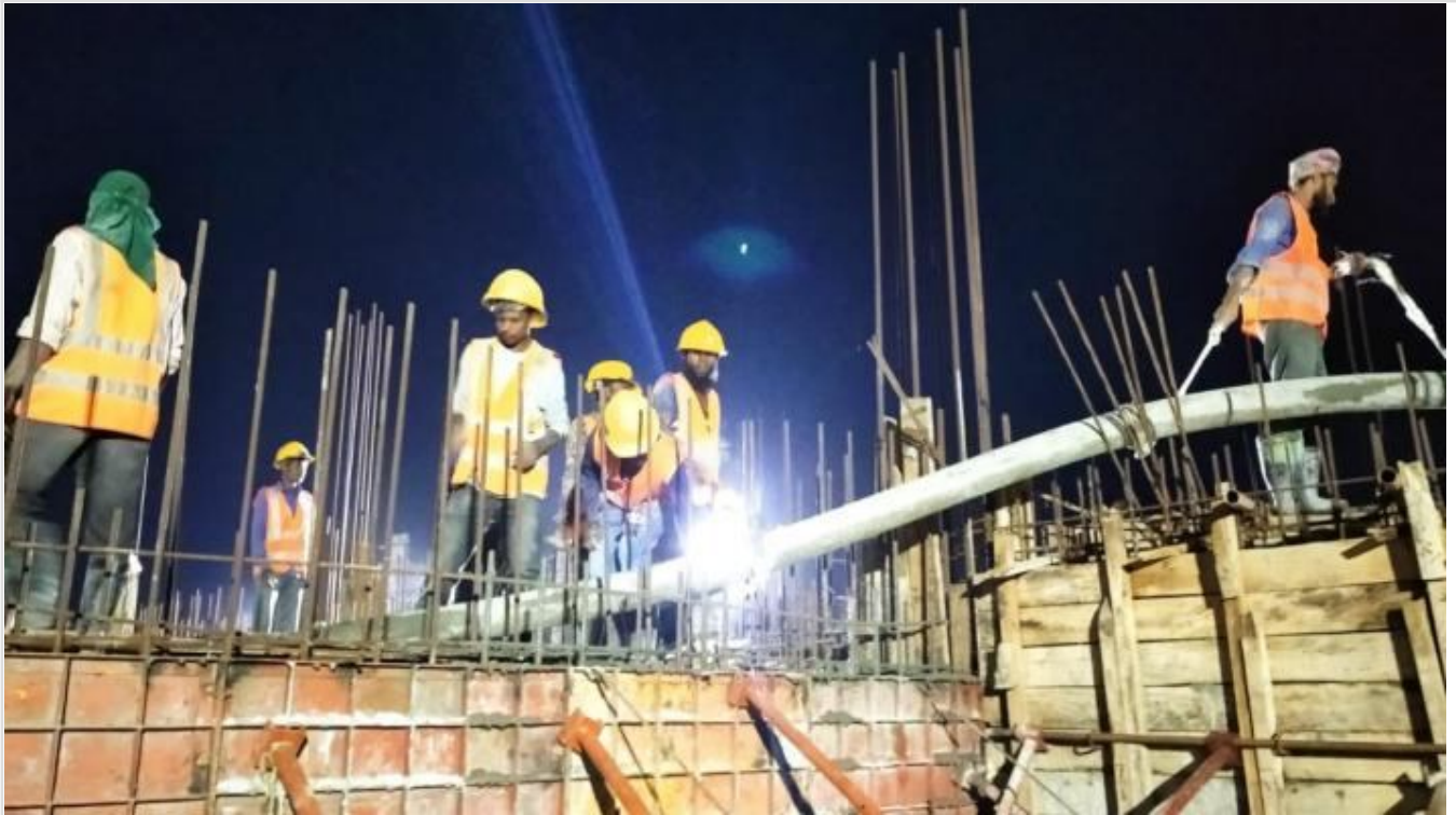
Water Reservoir Wall Concreting on 05-04-21
