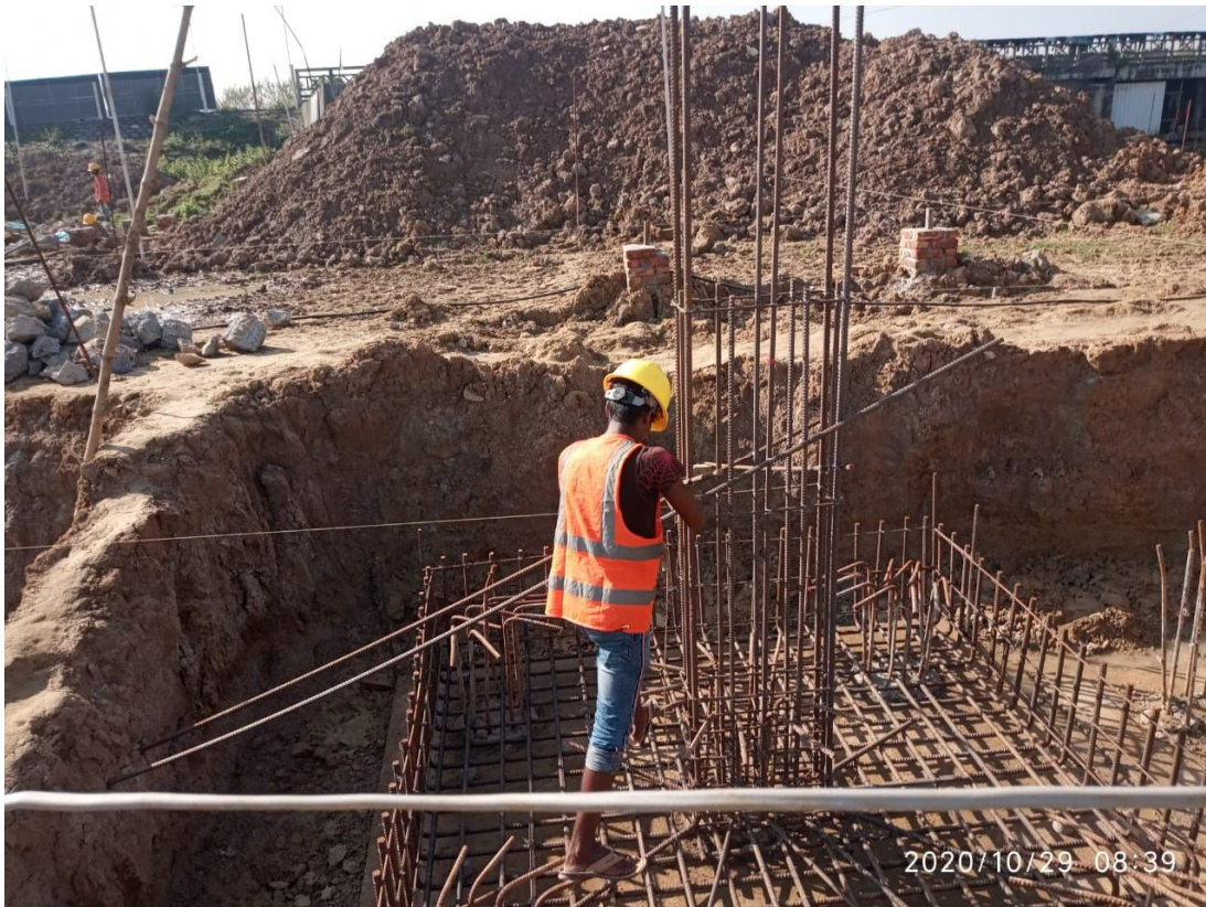
19 Oct 2020 : Pile Cap Re-bar work
