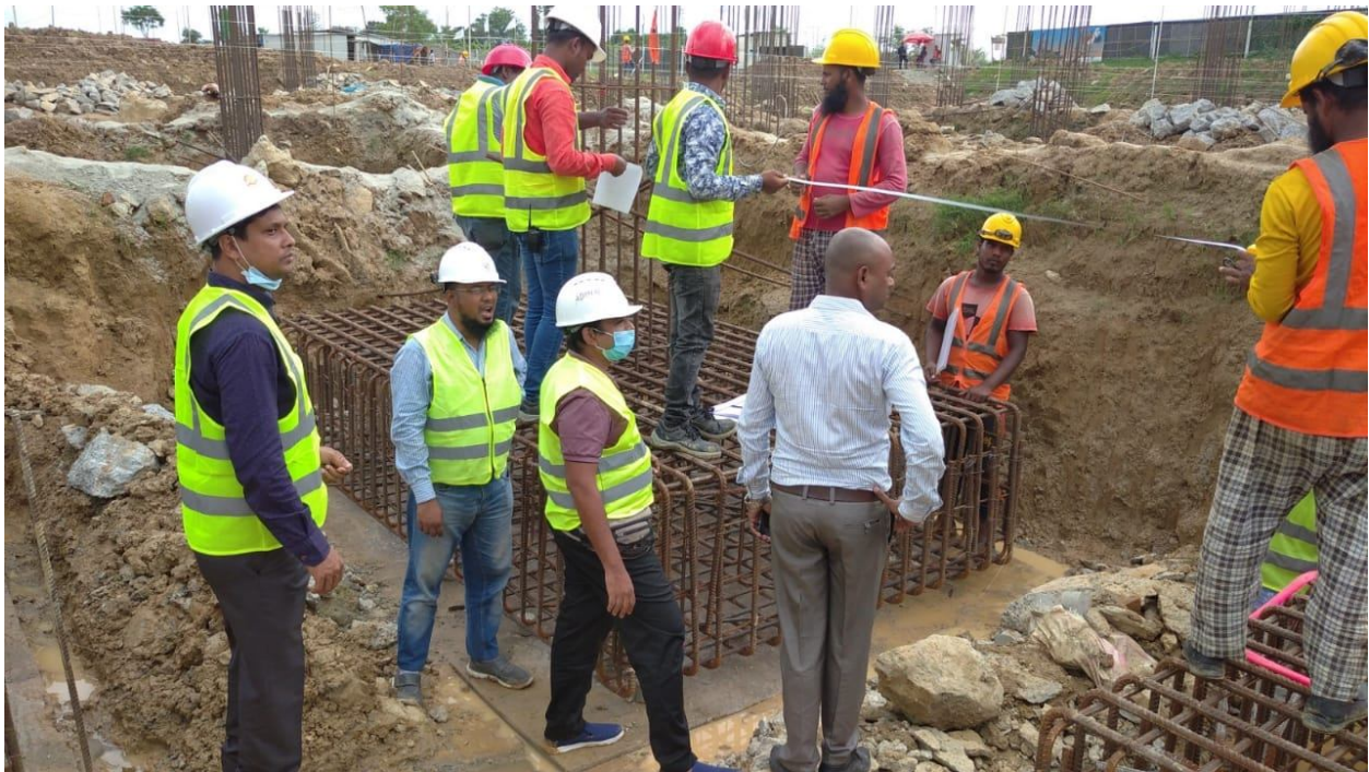
01 Nov 2020: Pile Cap Inspection before concreting
