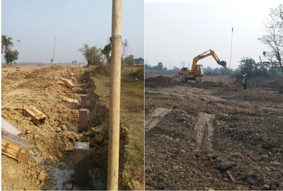
02 Mar 2020: Boundary Fencing Column
