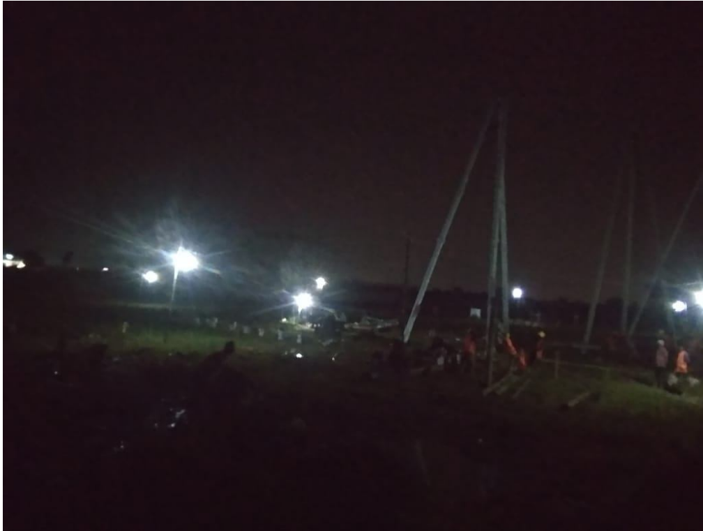
28 Aug 2020: Piling Work-night shift
