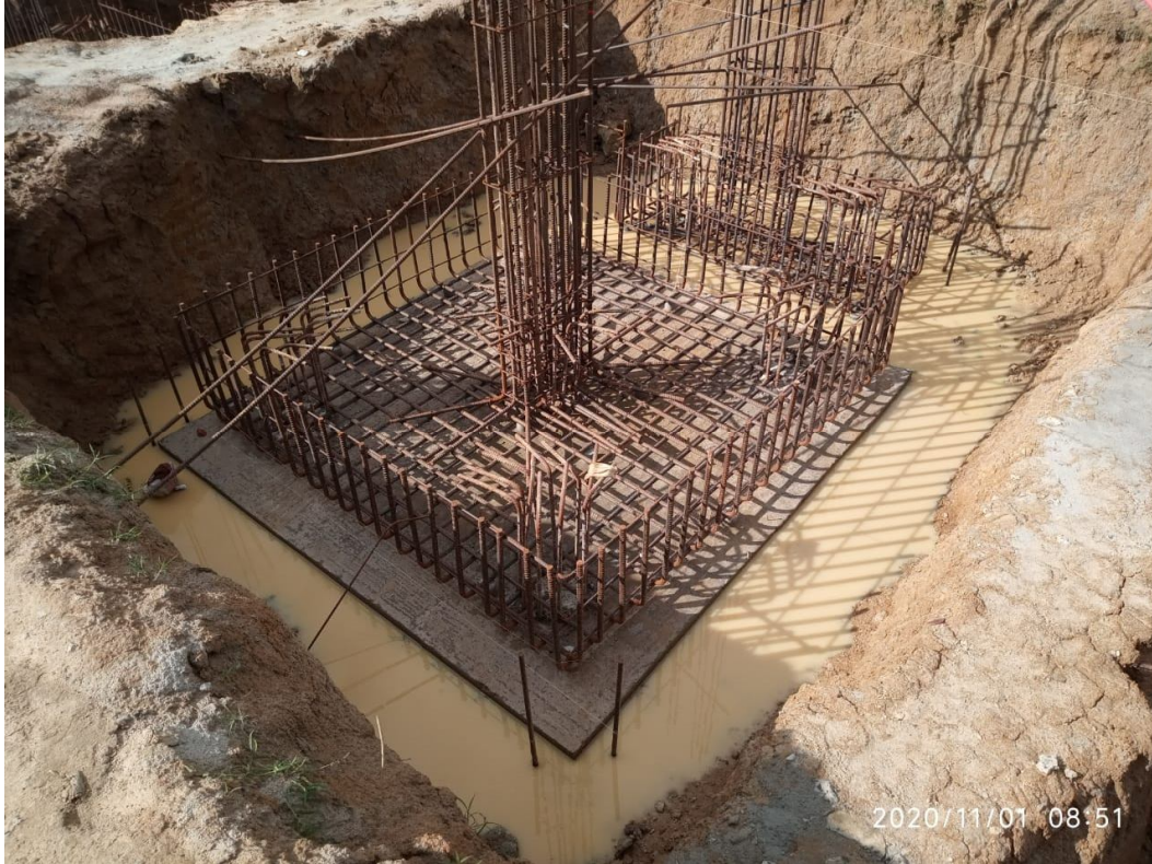
01 Nov 2020: Pile Cap
