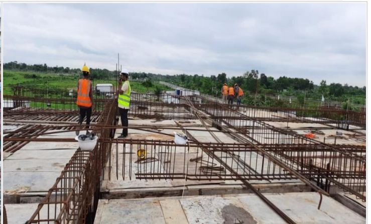
1st floor Slab Shuttering on 12-06-21
