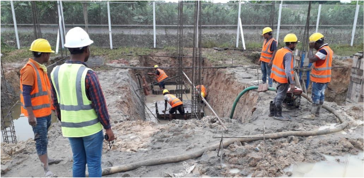
14 Sep 2020 : Sub-station Footing
