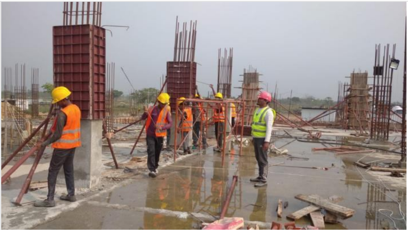
Column Shuttering on 10-04-21
