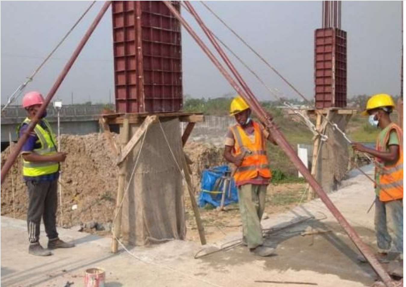
Column Shuttering on 09-05-21
