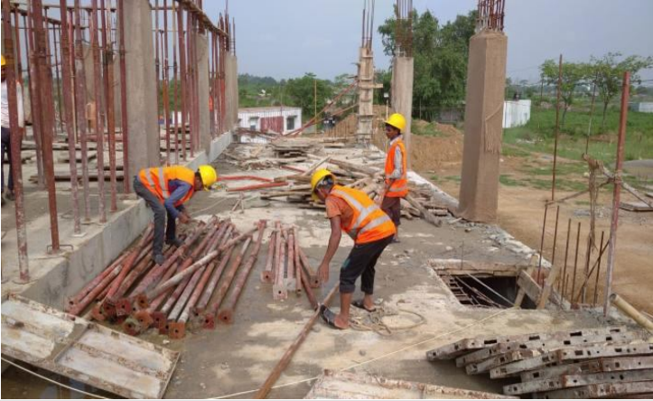
1st Floor Slab Shuttering on 03-06-21
