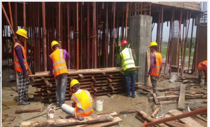
1st floor Slab Shuttering on 15-06-21
