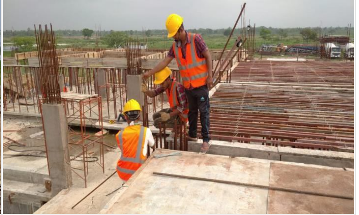
1st Floor Slab Shutter Levelling on 03-06-21
