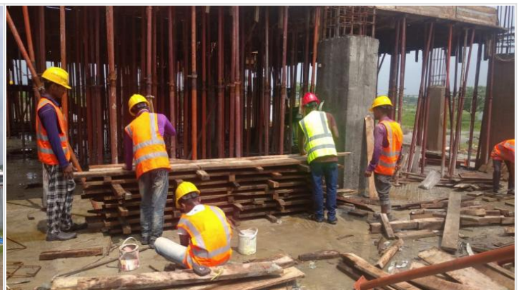
1st floor Slab Shuttering
