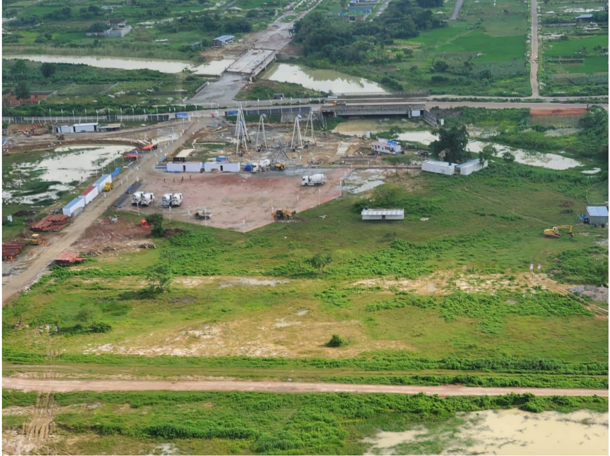
13 Sep 2020: Project View from Top
