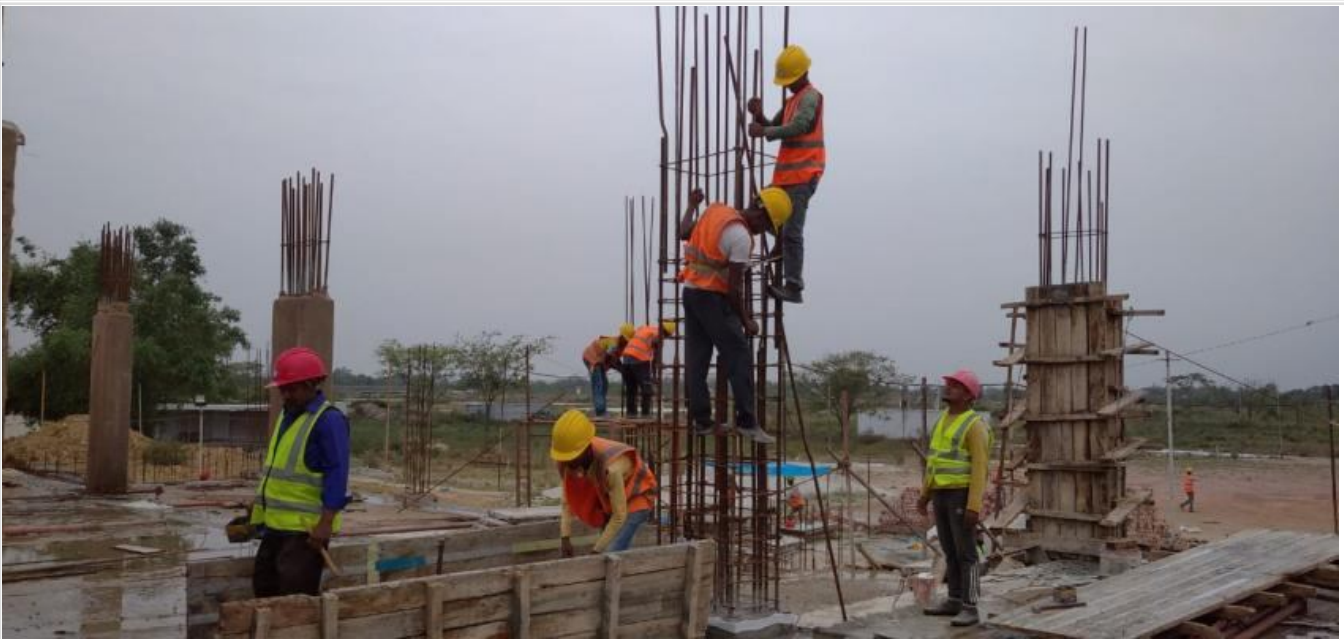
Column Re-bar Work on 08-05-21
