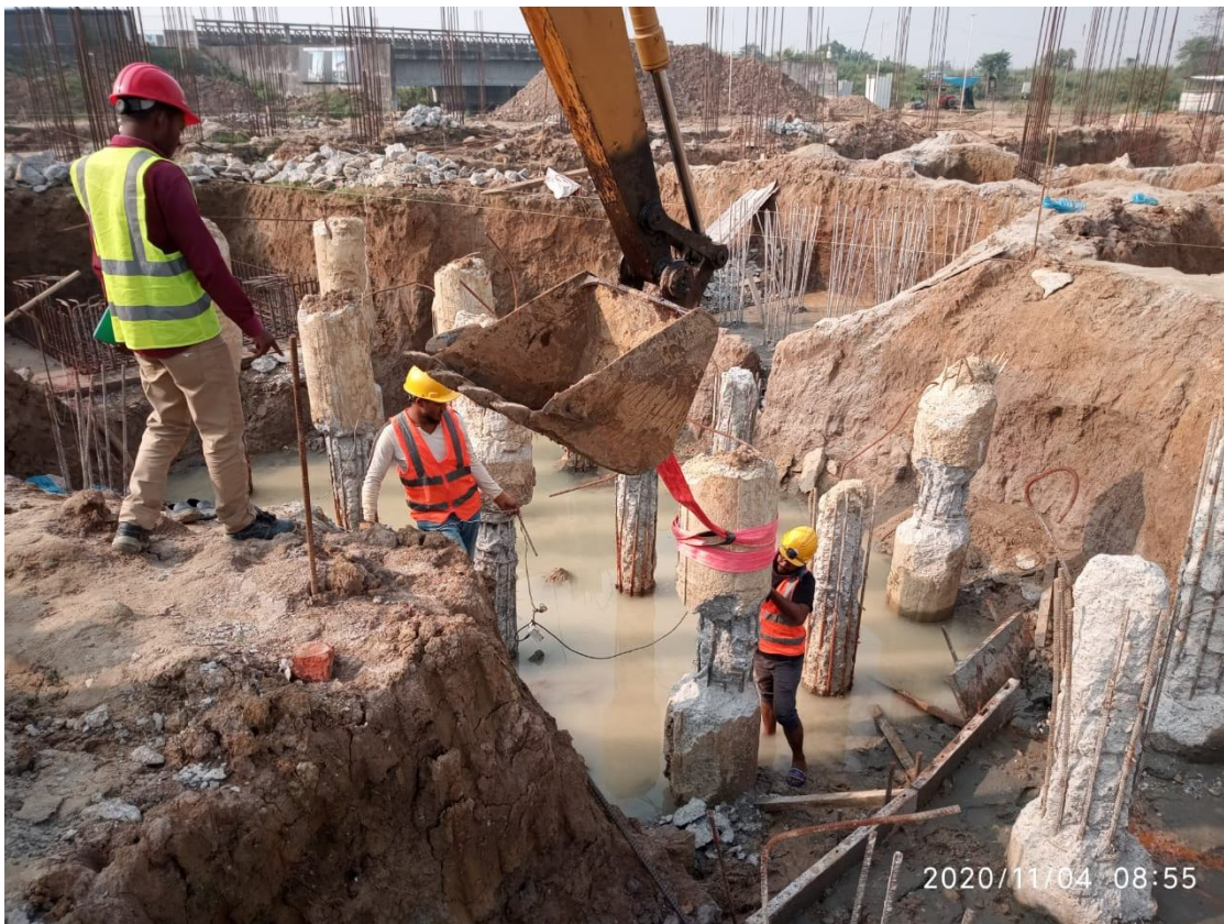
03-04 Nov 2020 : Pile Head Breaking, Pile cap re-bar
