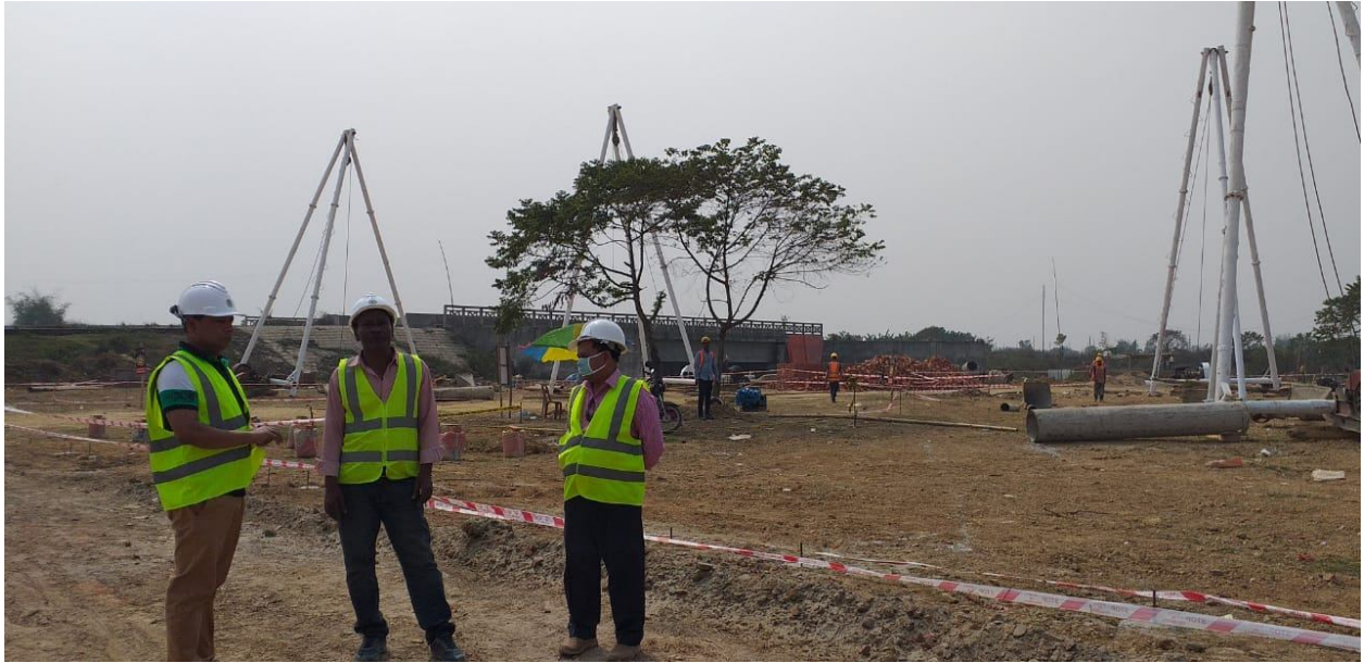
20 Feb 2020: Piling Rig
