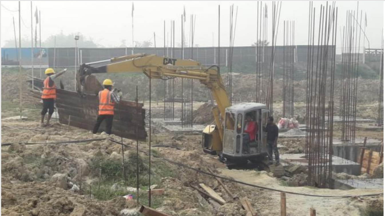
Pile Cap Re-bar Shuttering Work on 05-12-20
