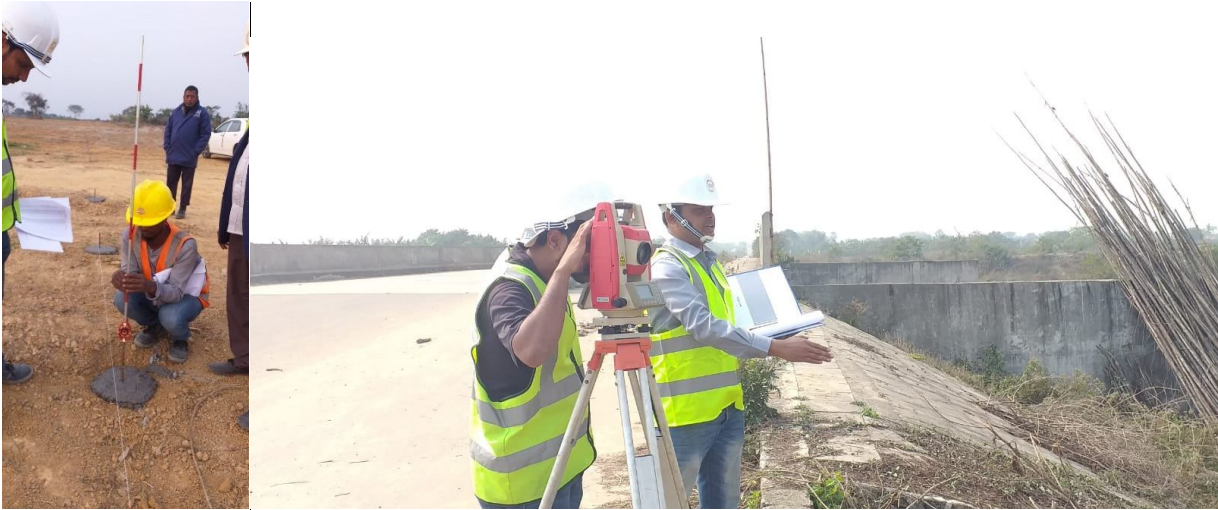
05 Feb 2020: Survey work
