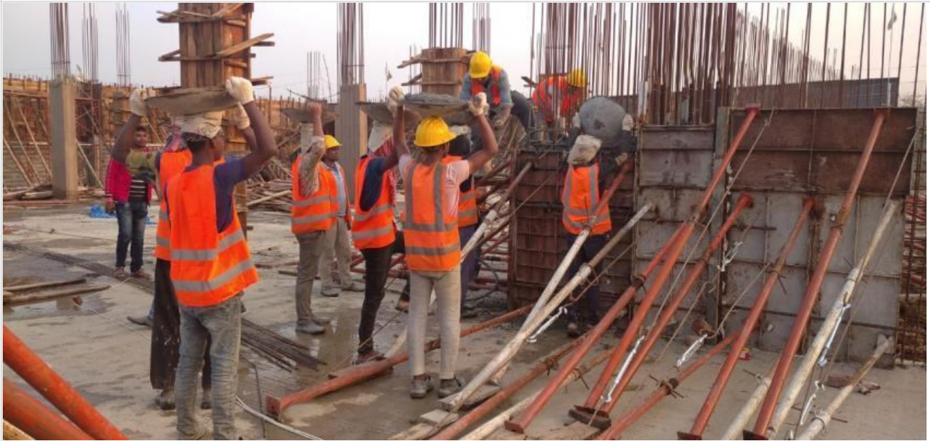
Retaining wall and Column Concreting on 28-01-21
