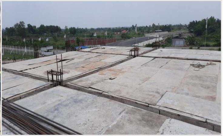
1st floor Slab Shuttering on 09-06-21
