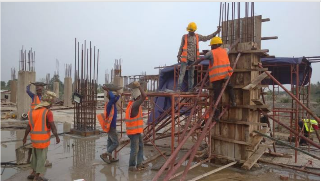
Column Re-bar Work on 04-05-21
