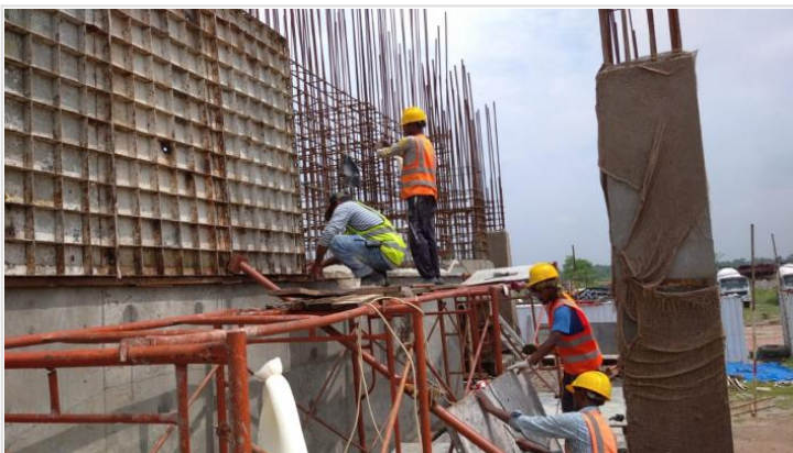
Ground Floor Lift Core Shuttering
