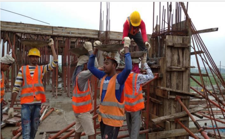
Ground Floor Column Concreting on 06-06-21
