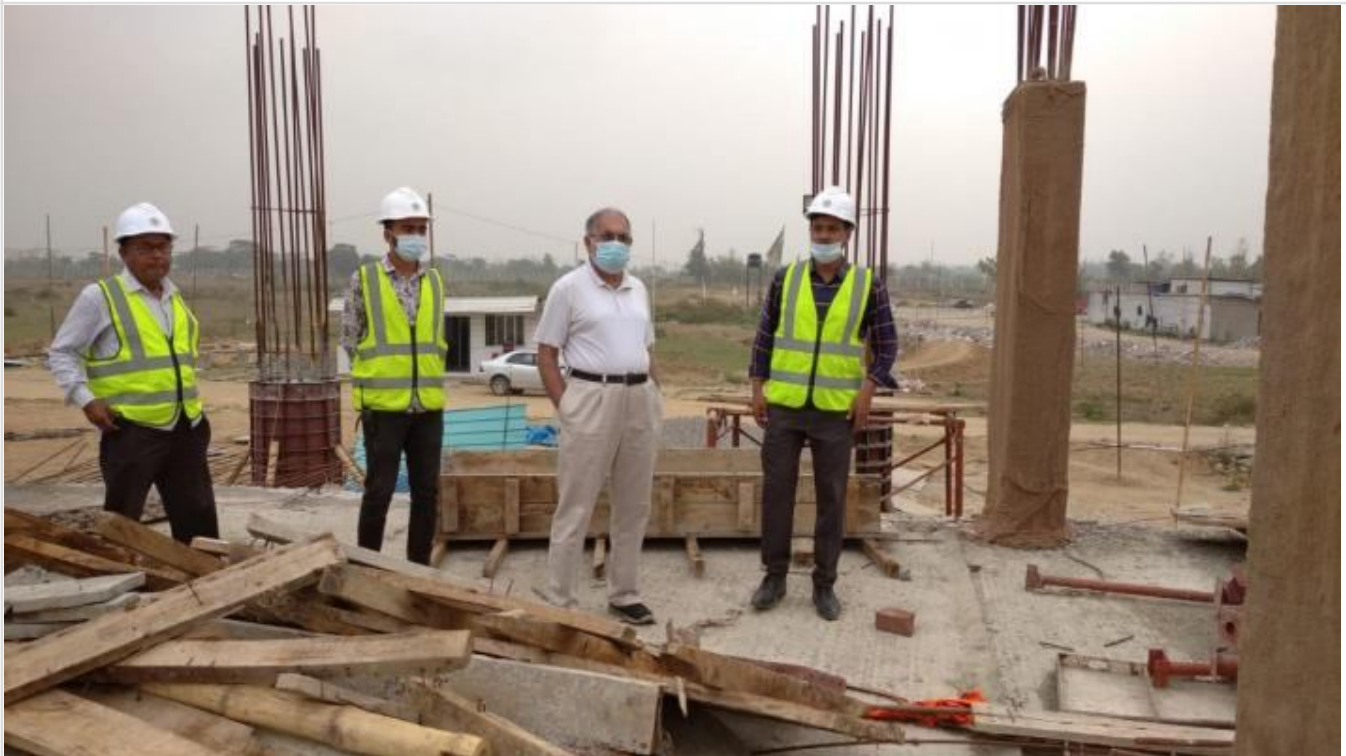
G.M. Construction Visit on 28-04-21
