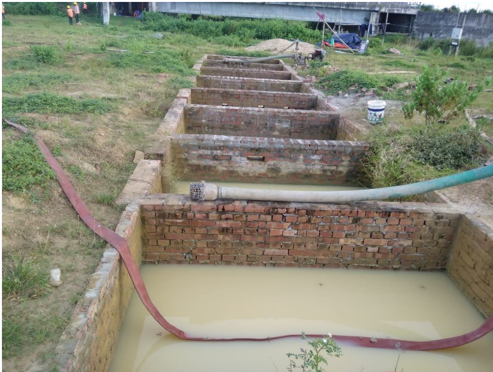
25 Aug 2020: Pile Mud Tank
