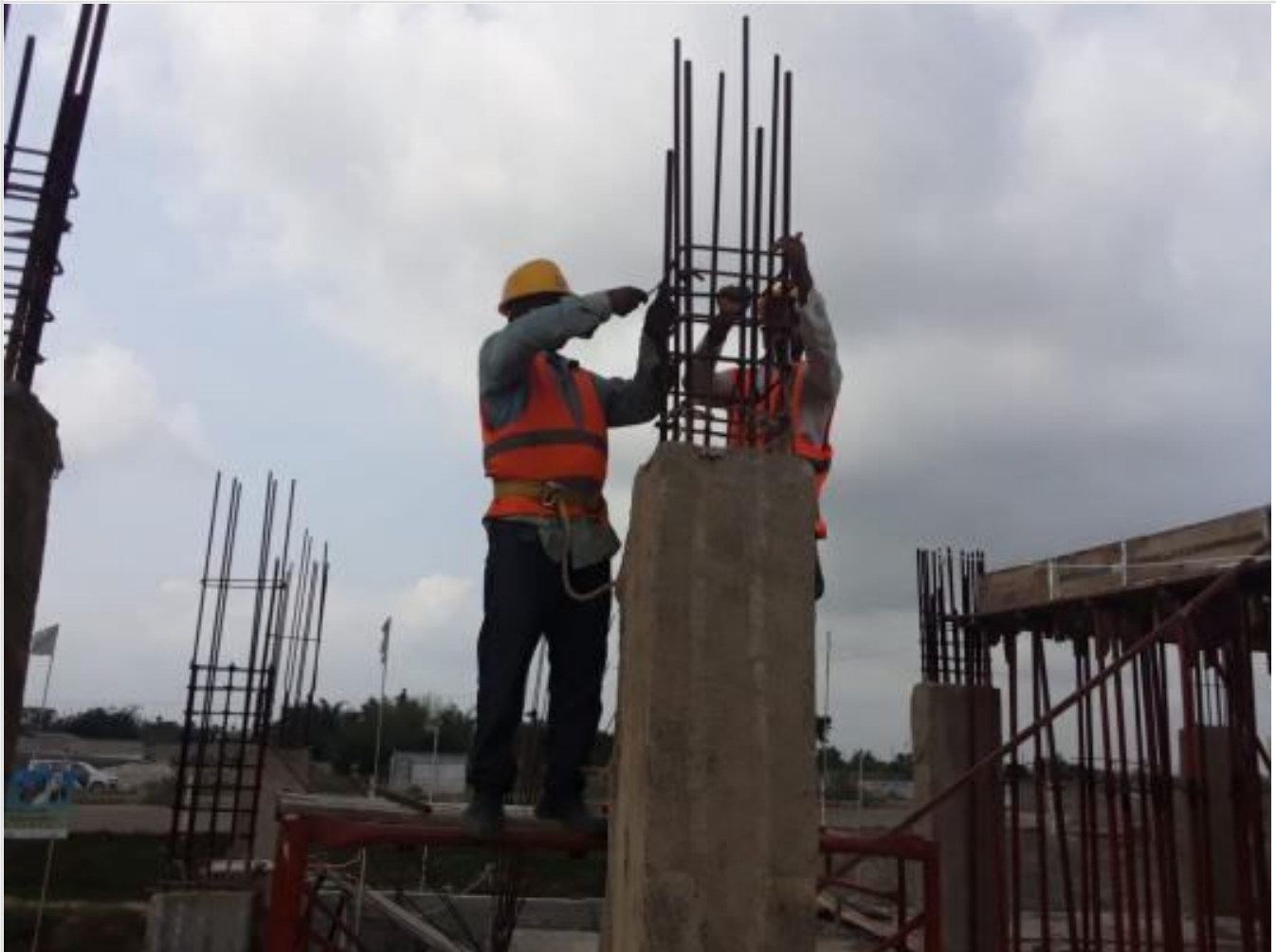
Ground Floor Re-bar Work on 20-05-21
