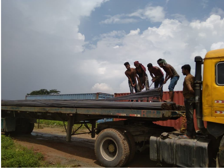
28 Aug 2020: Pile Re-bar
