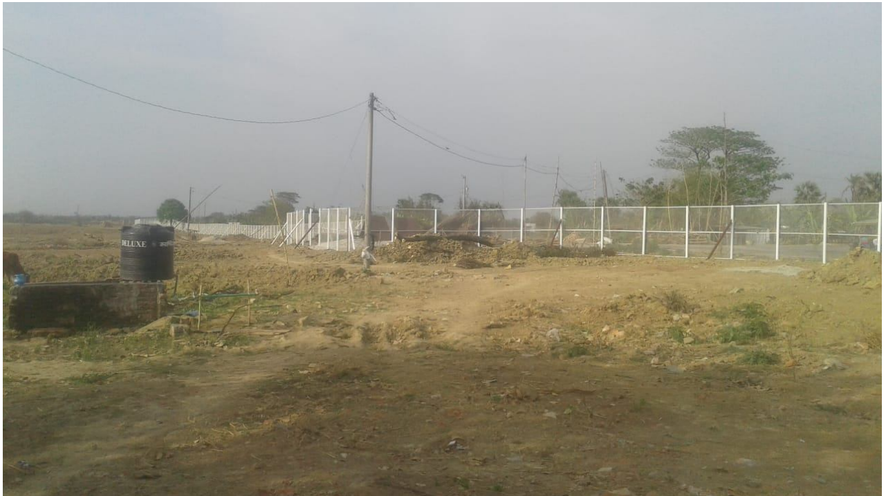
01 Apr 2020 : Boundary Fencing
