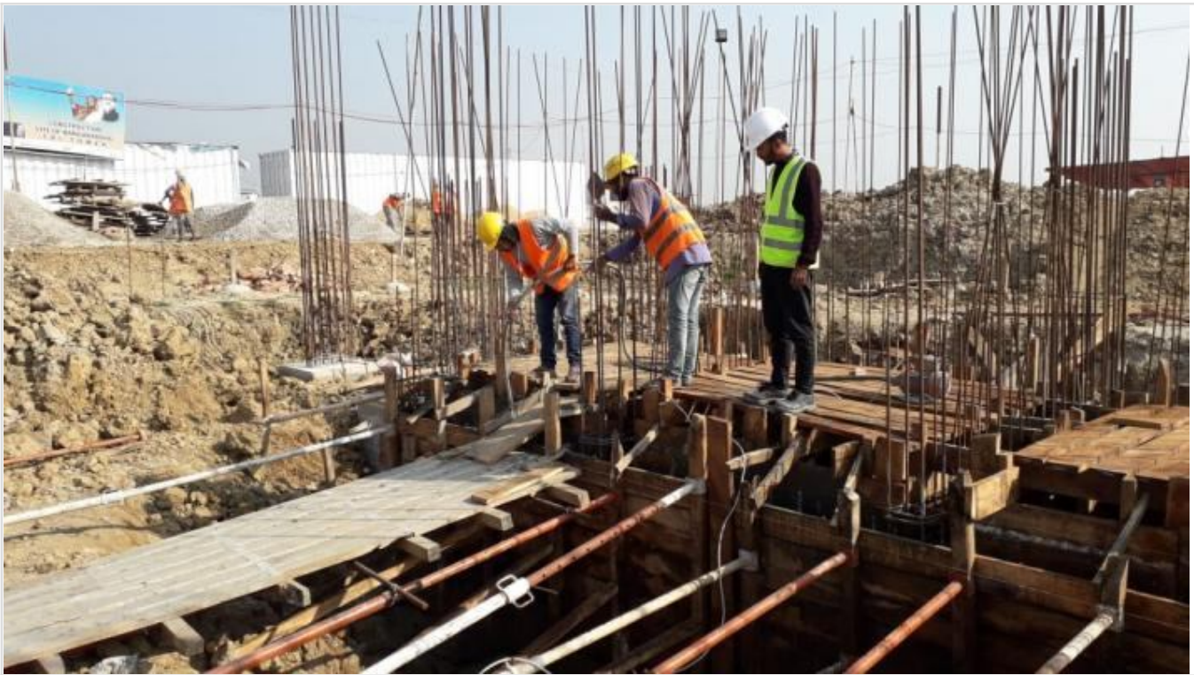
Lift Core Concreting on 19-12-20
