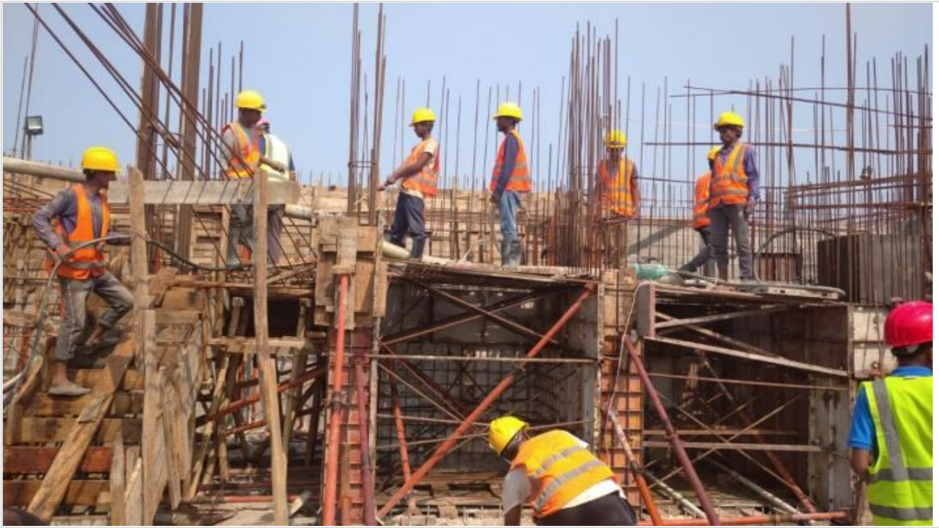
Lift Core Wall Concreting on 05-04-21
