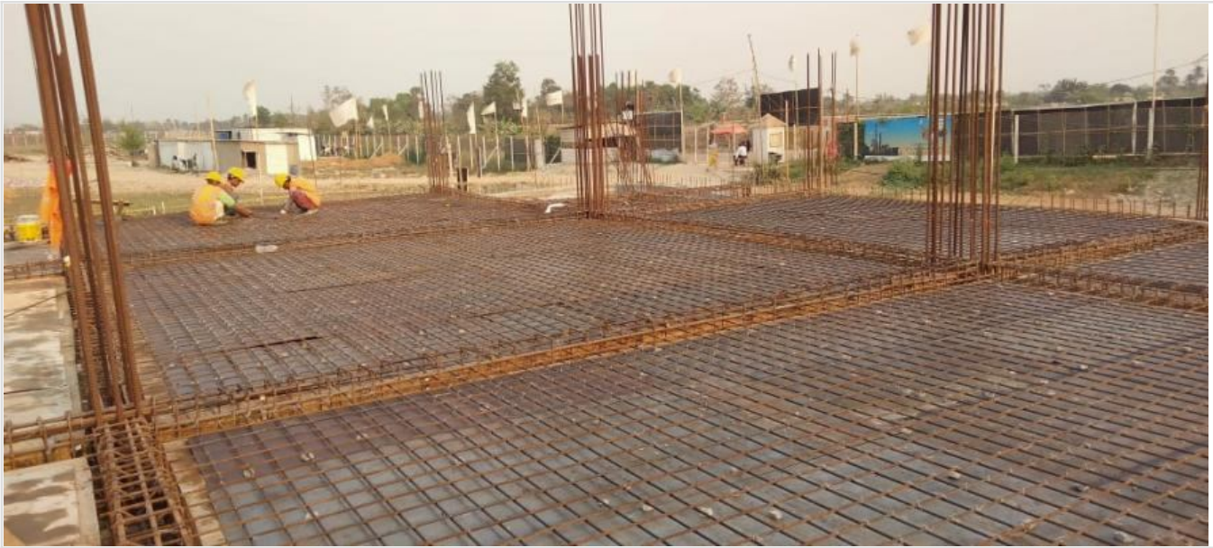
Ground Floor Slab Re-bar Work on 10-03-21
