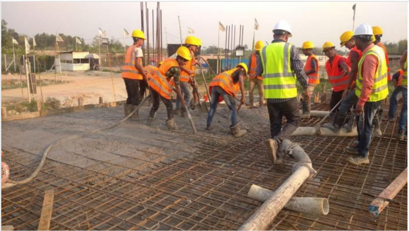
GF North-Slab 8000 sft Concreting on 15-03-21
