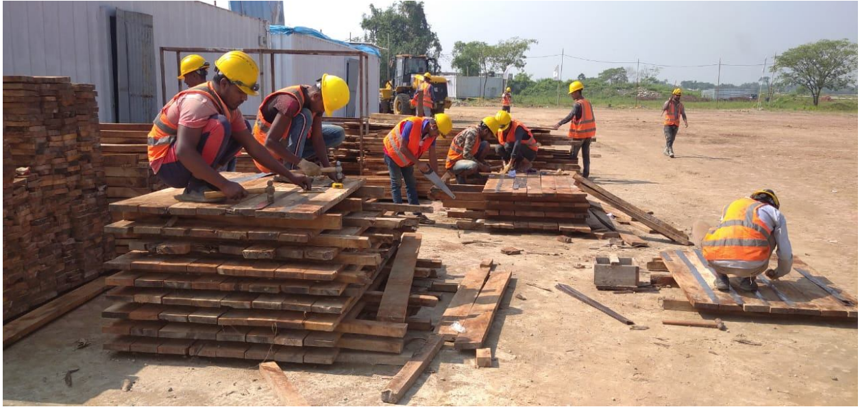
05 Nov 2020: Pile cap shutter making
