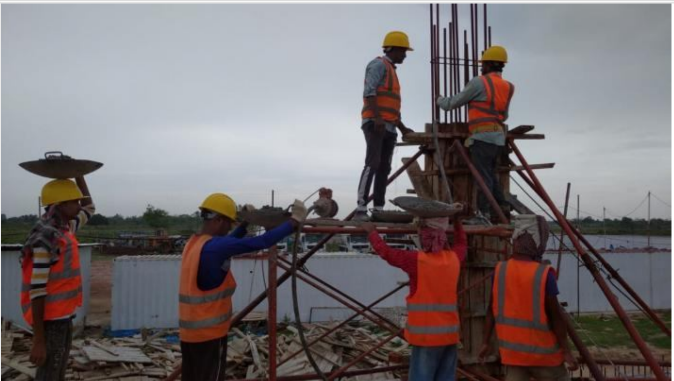
Ground Floor-Column Concreting on 26-05-21
