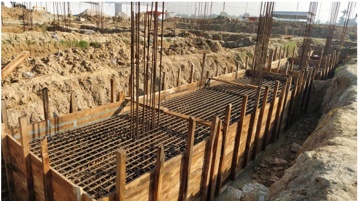
16 Nov 2020: Pile cap shutter fixing
