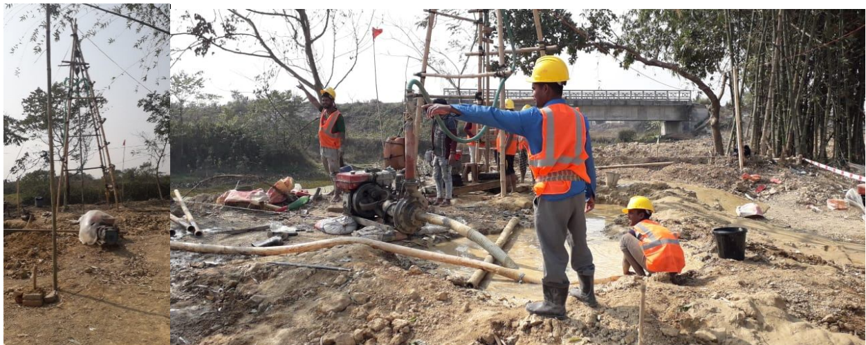
10-13 Feb 2020 : Tube well Sinking
