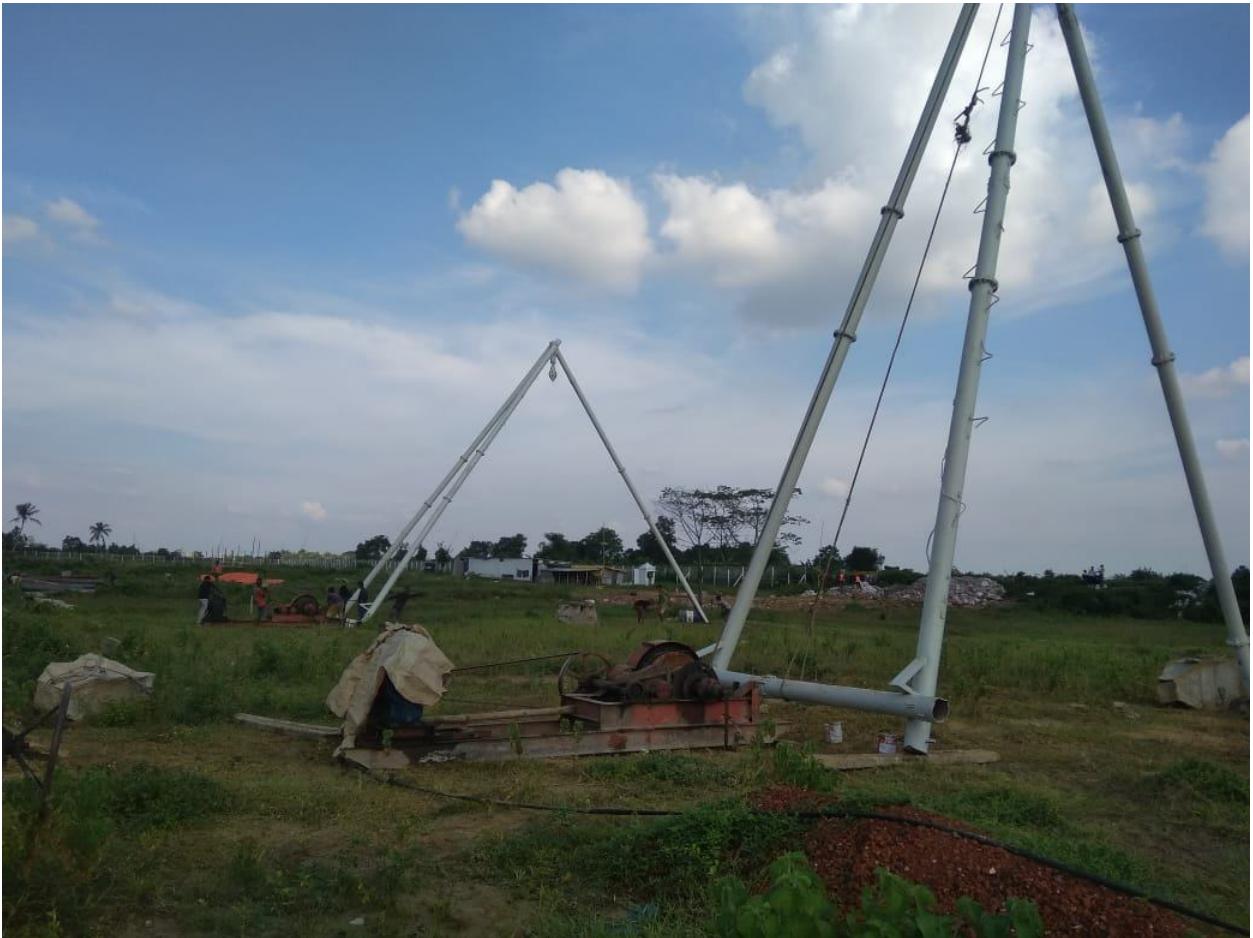
24 Aug 2020: Piling Rig Installed
