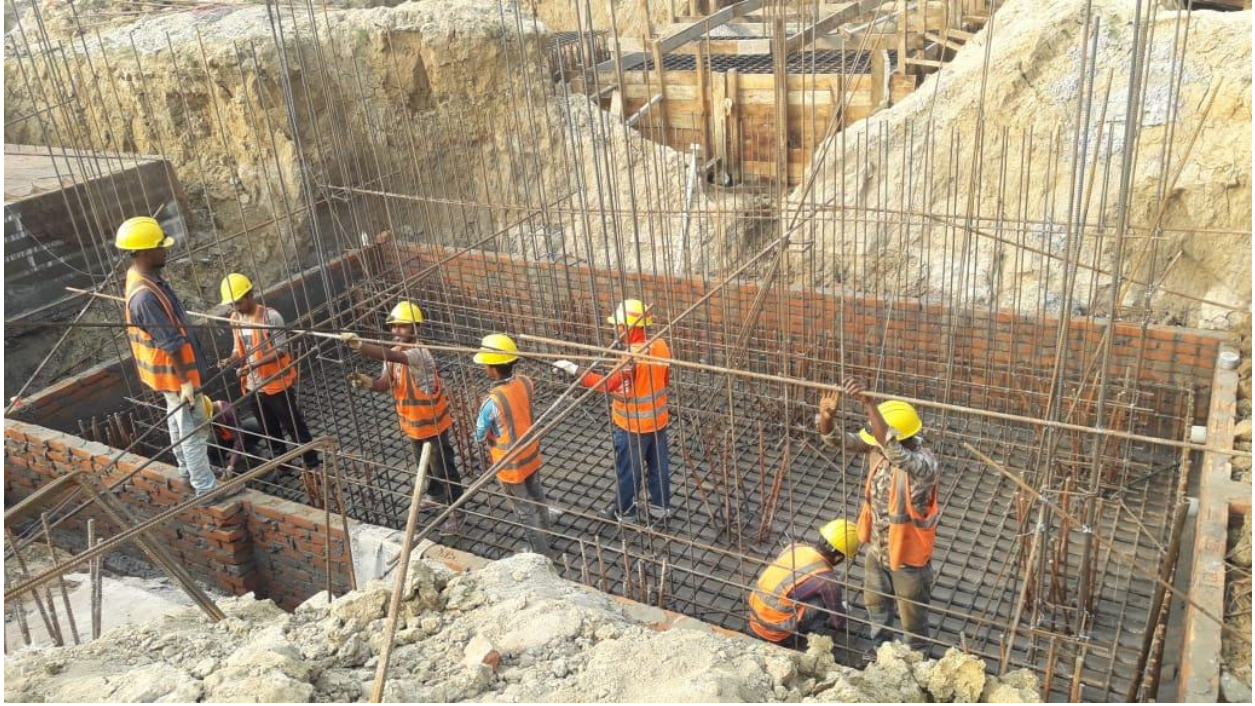
03 Dec 2020 : Brick wall for Shuttering
