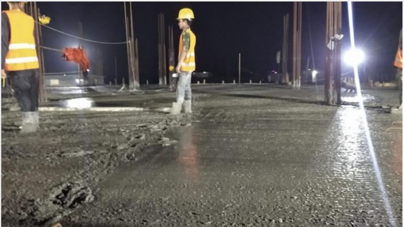
GF Slab Concreting complete at night on 15-03-21
