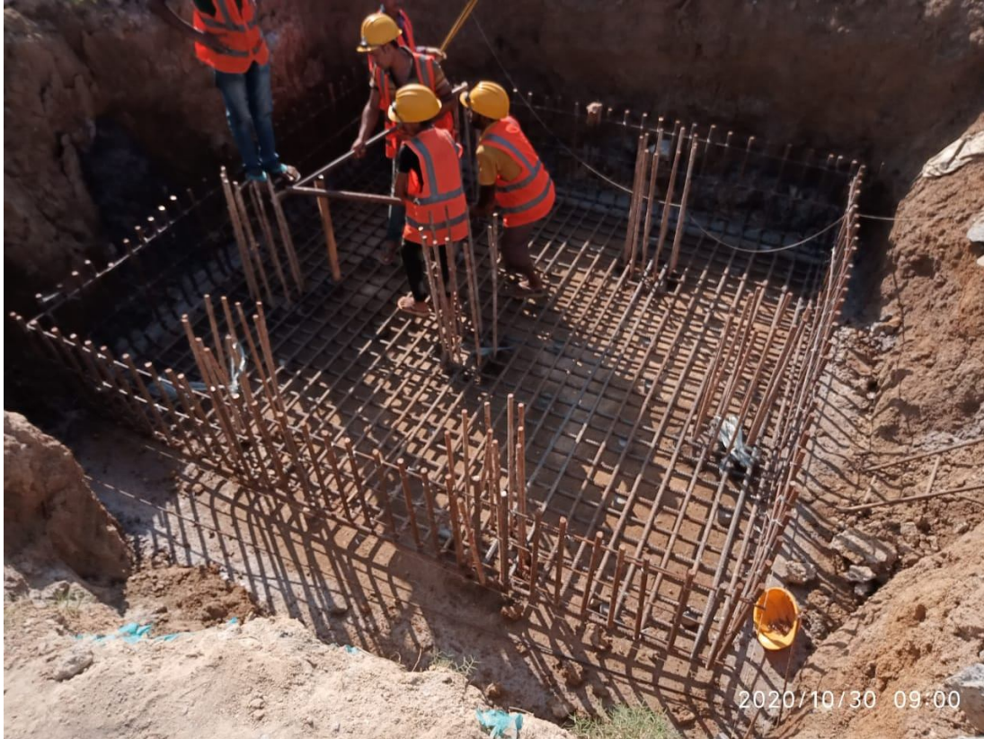
30 Oct 2020: Pile Cap Re-bar work
