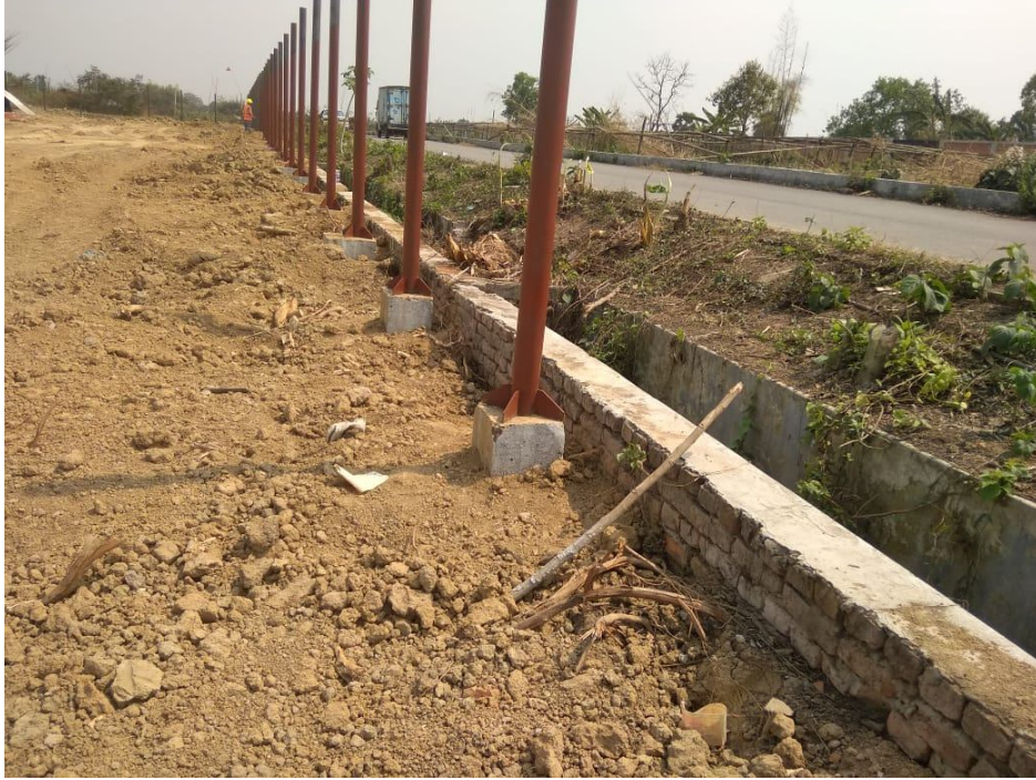
03 Mar 2020: Boundary Fencing Column
